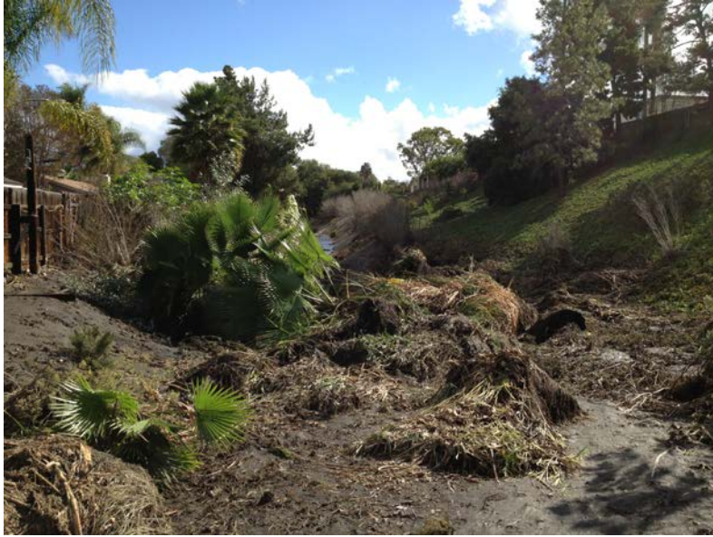
Photo 1. General condition of the San Carlos Channel and adjacent area, on 11/1/2014 after initial storm, prior to work beginning and prior to second storm began.
