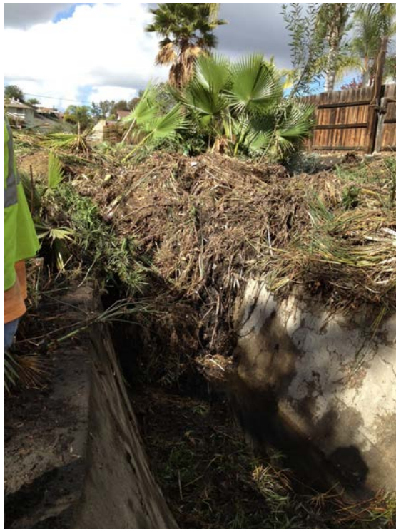
Photo 2. Condition of opening to culvert on 11/1/2014 after initial storm, prior to work beginning and prior to second storm began.
