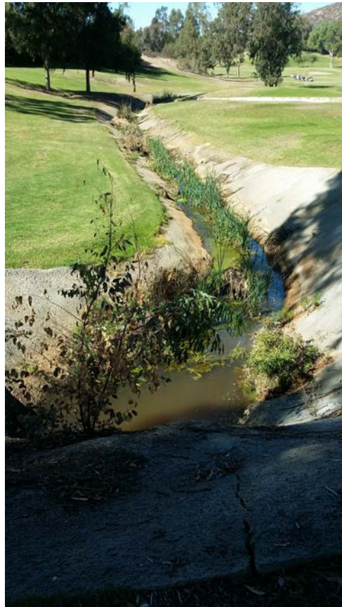
Photo 5. Condition of channel east of Cowles Mountain Blvd prior to emergency, 10/30/2014, looking west of culvert.
