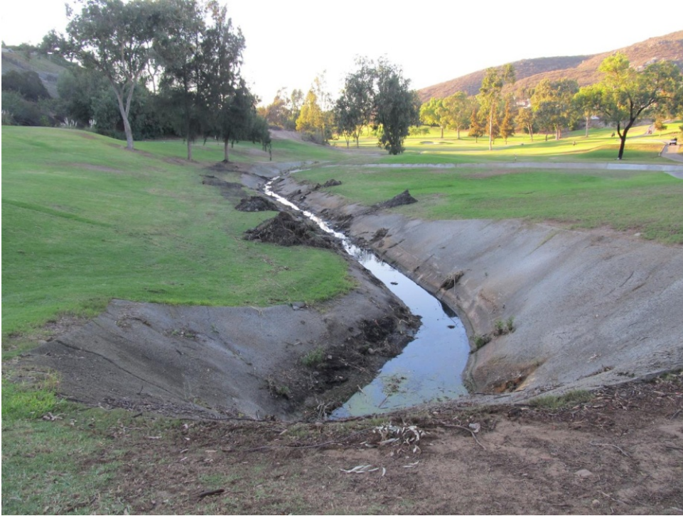
Photo 7. Condition of channel west of Cowles Mountain Blvd after emergency maintenance activities commenced.
