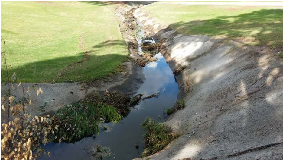
Photo 6. Condition of channel west of Cowles Mountain Blvd after rain event on 11/1/2014, prior to emergency maintenance commencing.
