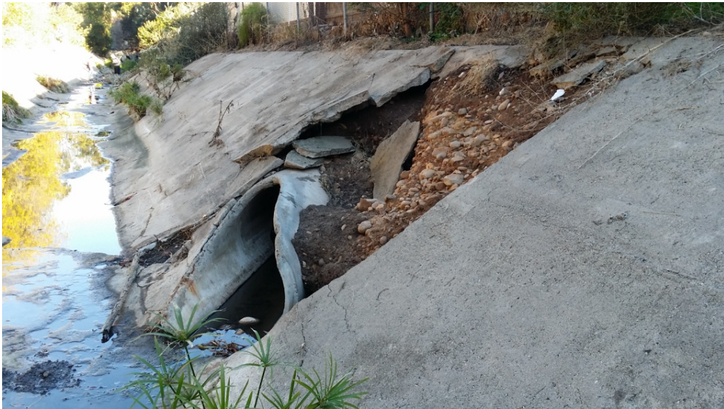
Photo 3. Condition of upstream portions of San Carlos Channel on 11/6/2014 after rain event. Note the concrete panels that have broken off and washed down into the channel.
