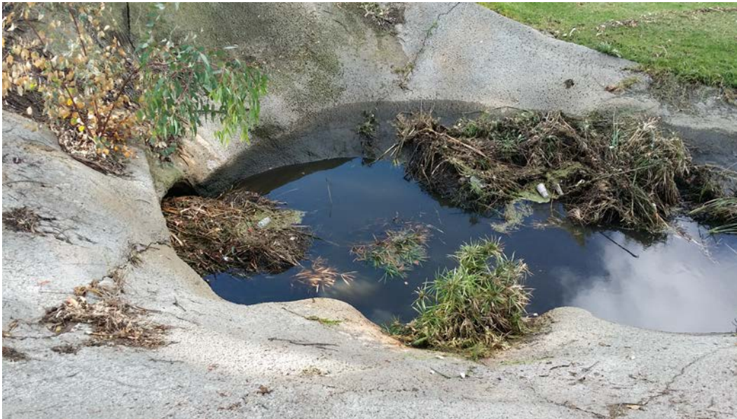
Photo 4. Condition of channel east of Cowles Mountain Blvd after first rain event on 11/1/2014, prior to emergency maintenance commencing, looking at outlet to culvert.
