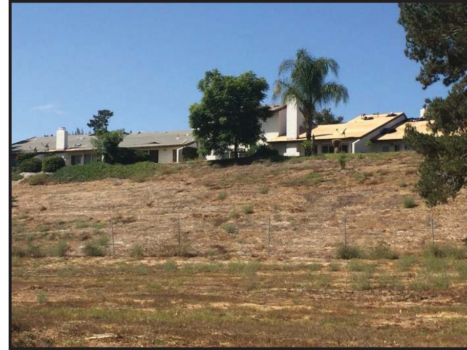
9. Photograph showing another view of fuel modification being conducted along west edge of property.
