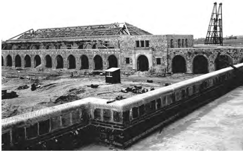
Figure 6: Marine Corps Recruit Depot under construction. Source: http://www.sandiegohistory.org/timeline/images/6917.jpg
