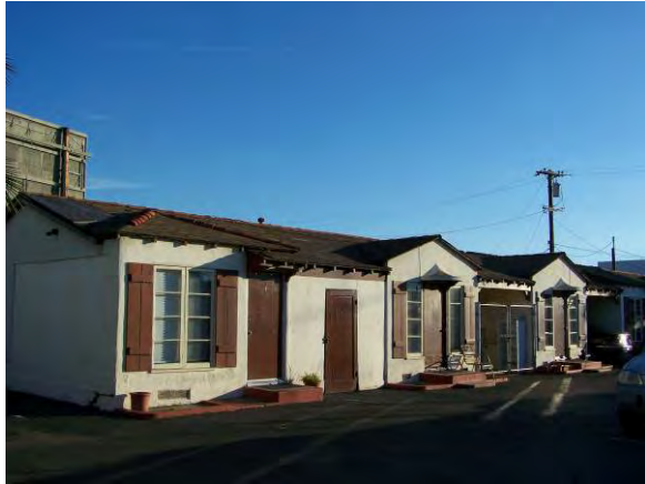
Figure 15: Twin Palms Motor Hotel, 4430 Pacific Highway
