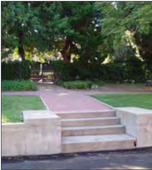
Figure F.19: Retaining Wall/Stairs at Street.
