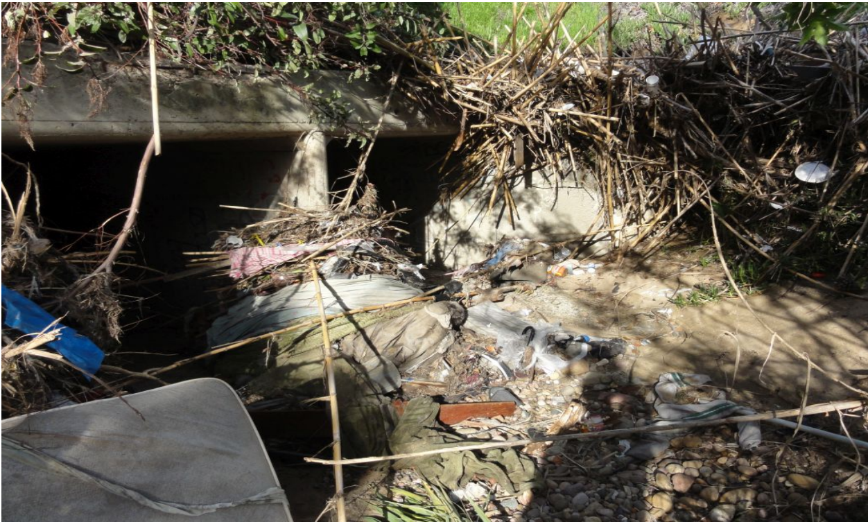
Downstream portion of Auburn Creek Channel Reach 1 facing west (downstream). Photo shows 50% clogging of box culvert. No flowing water was observed in Reach 1.
