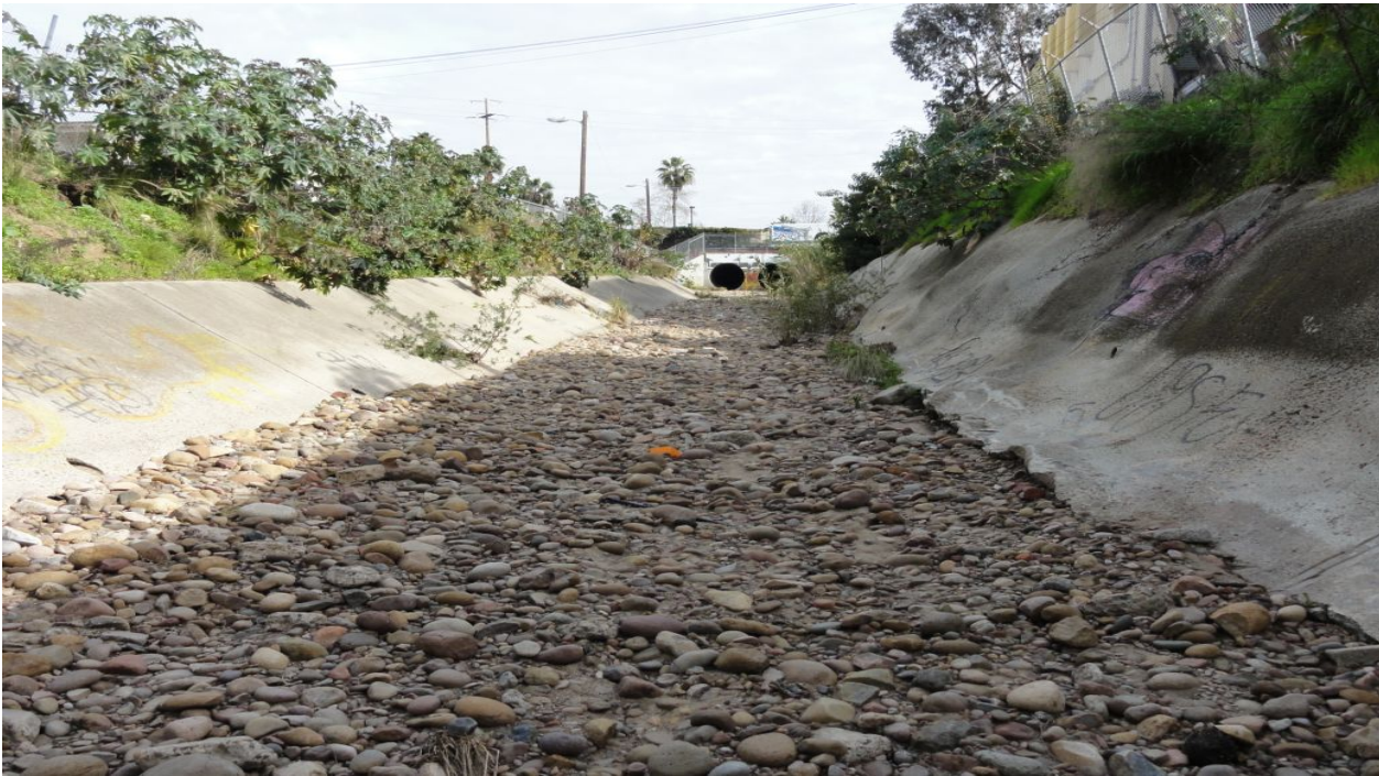
Middle portion of Auburn Creek Channel Reach 5 facing northeast (upstream). No flowing water was observed in Reach 5.
