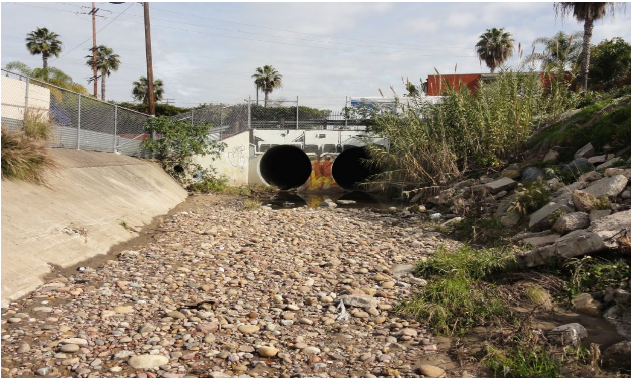
Upstream portion of Auburn Creek Channel Reach 5 facing northeast (upstream) at the 74'' double concrete pipe culvert. No dry weather flows and ponded water was observed in Reach 5.
