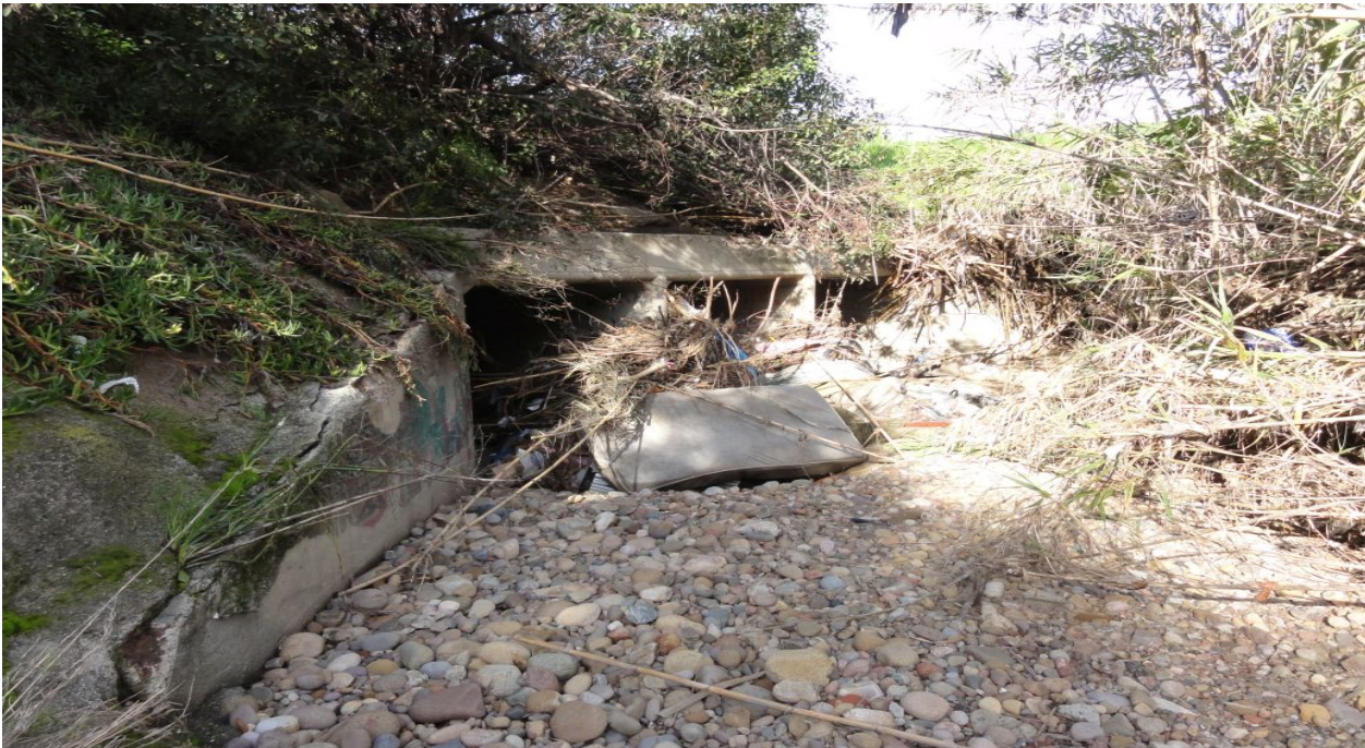
Downstream portion of Auburn Creek Channel Reach 1 facing west (downstream) at the triple 6-ft. by 6-ft. box culvert under Spillman Drive. No flowing water was observed in Reach 1.
