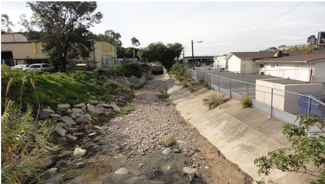
Auburn Creek Channel Reach 5 facing southwest (downstream). No dry weather flows and ponded water was observed in Reach 5.
