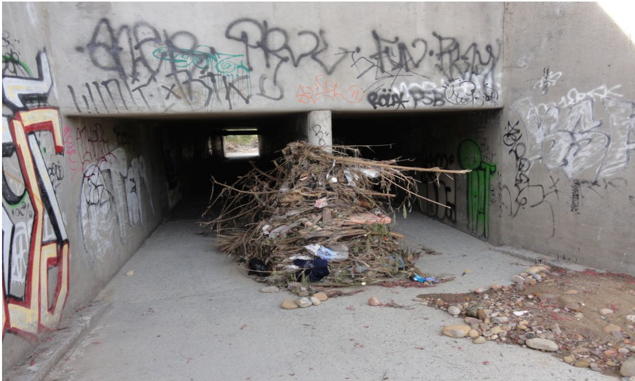
Downstream portion of Auburn Creek Channel Reach 5 facing southwest (downstream) at the 6-ft. by 6-ft. double box culvert. No flowing water was observed in Reach 5.
