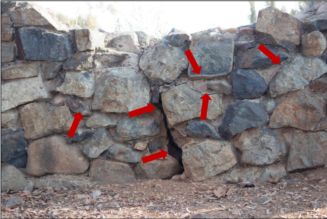
Figure 7. Detail view of wall section showing missing portions and cracks (red arrows).
