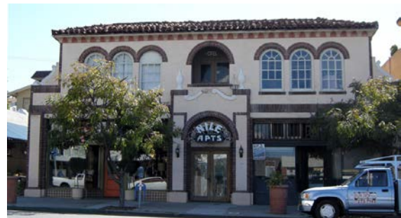
Nile Apartments, 3791 Park Boulevard.
