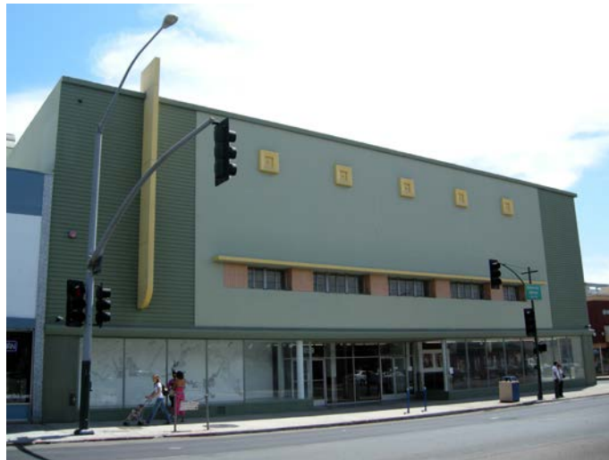
J.C. Penney Co. Building, 3029 University Avenue.
