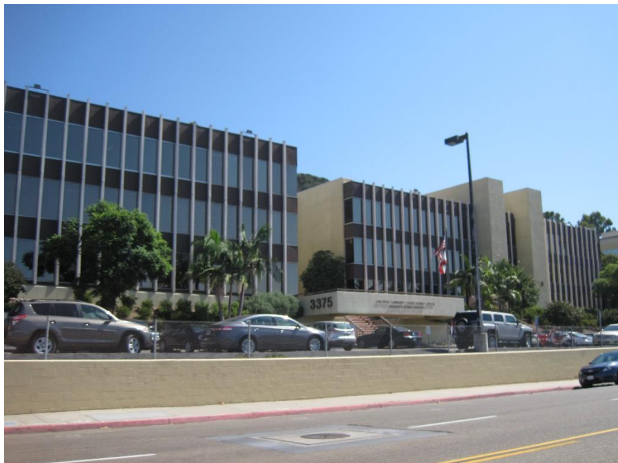
Figure 3-26: San Diego Community College District Offices at 3375 Camino del Rio South. Note the building's symmetrical composition, simple geometric form, flat roof, clear expression of structure and materials, and large expanses of glass.
