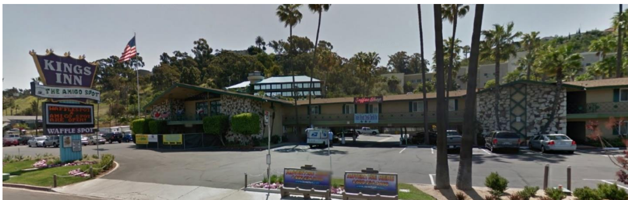
Figure 3-23: Kings Inn at 1333 Hotel Circle South.
