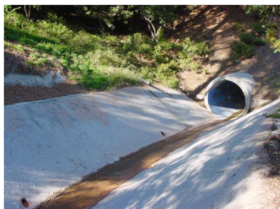
City of San Diego storm drain
