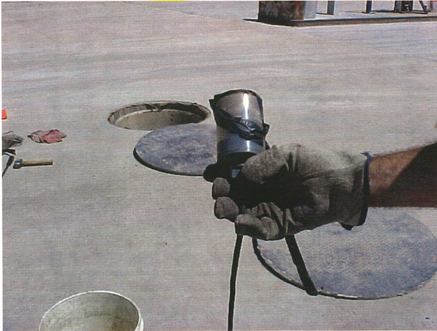
Annular space sensor in the T-2 (HMD's T004) south diesel tank is being held together by electrical tape.
