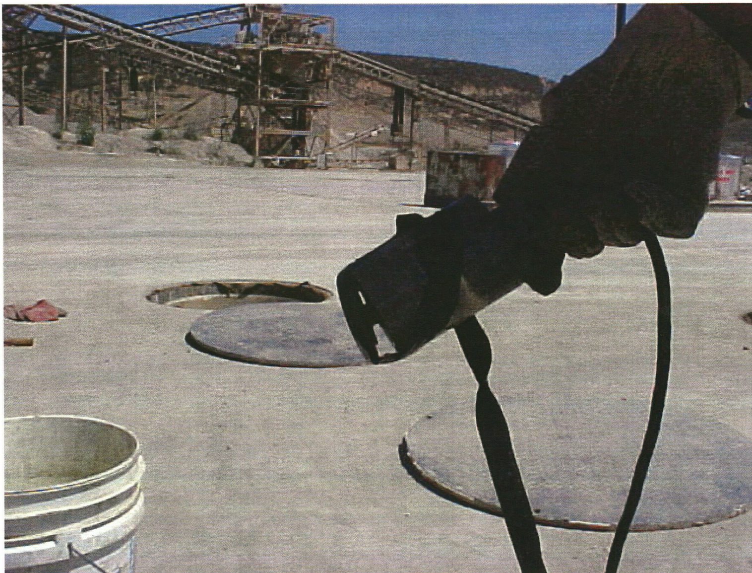
Annular space sensor in the T-2 (HMD's T004) south diesel tank is being held together by electrical tape.
