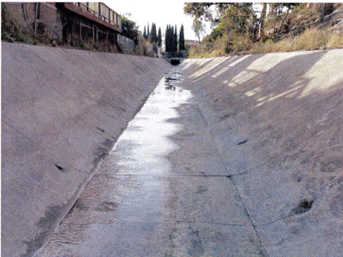
Photograph 11: Downstream view to culvert of Via de la Bandola channel after emergency maintenance.
