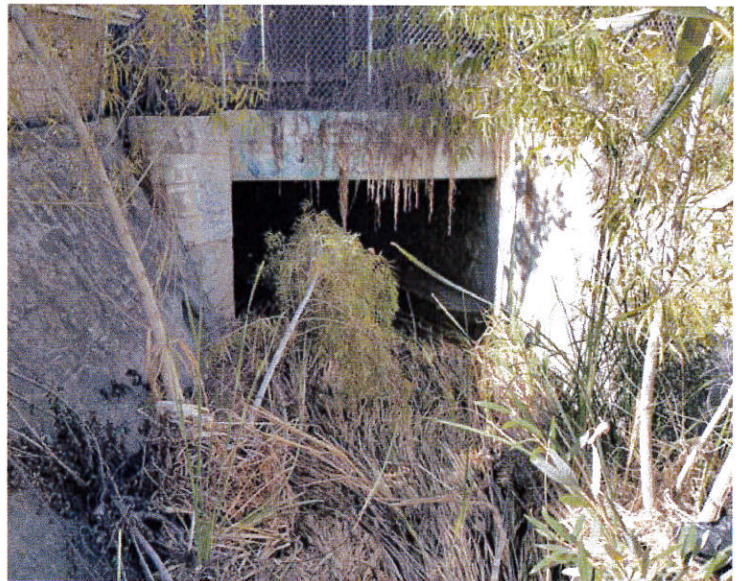
Photograph 8: Looking west in the channel to the culvert. 3094 Via de la Bandola is located above on the left.
