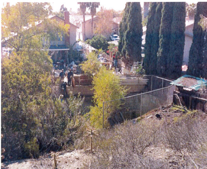
Photograph 9: On the north side of the channel looking south to 3094 Via de la Bandola and the culvert.
