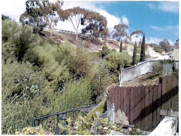
Photograph 4: Channel from equipment access looking east along channel from 4004 Via de la Bandola.
