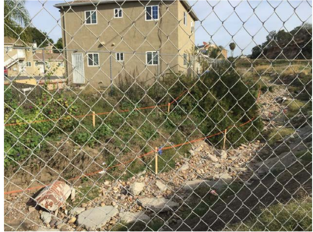
PHOTO 5: Looking upstream (EAST) standing directly above northerly box culvert. Staff is standing at the toe of slope. Removal of sediment will stop outside of the toe of slope and be level with the bottom floor of the channel. Area within orange tape will require the removal of sediment and vegetation.
