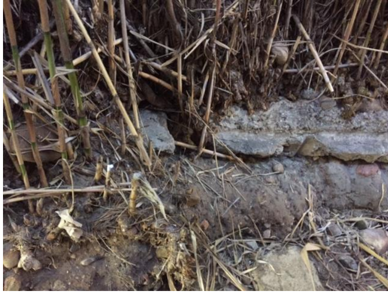
Photograph 9: Evidence of flooding damage compromising adjacent 5017 Wightman St. property footing within Proposed Impact Area Section 2 in MMP Map 68; Figure 3b.
