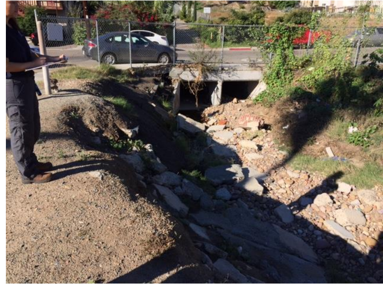
Photograph 13: Looking west toward Auburn Drive at the current sediment build up and clogging of right side of two-box culvert within Proposed Impact Area Section 3 in MMP Map 68; Figure 3b.
