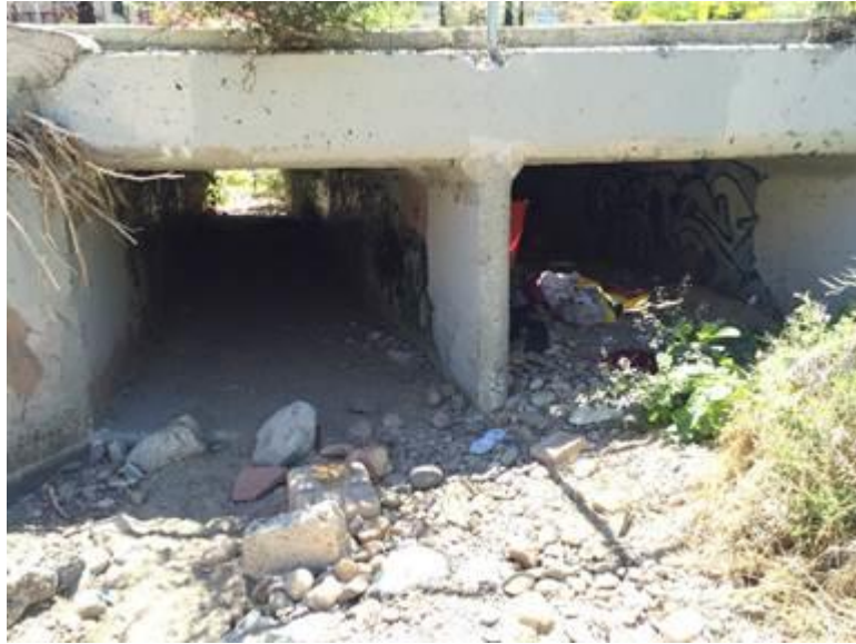
Photograph 13: Looking west toward Auburn Drive at sediment build up and clogging of right side of two-box culvert on May 20, 2015 within Proposed Impact Area Section 3 in MMP Map 68; Figure 3b.
