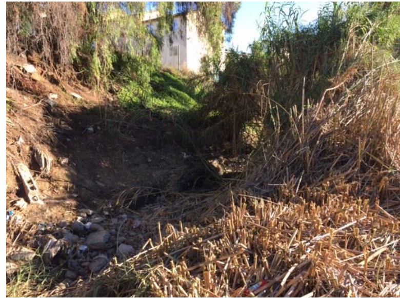
Photograph 4: Looking upstream at sediment and vegetation build up along channel on north end of MMP Map 67; Figure 3a.
