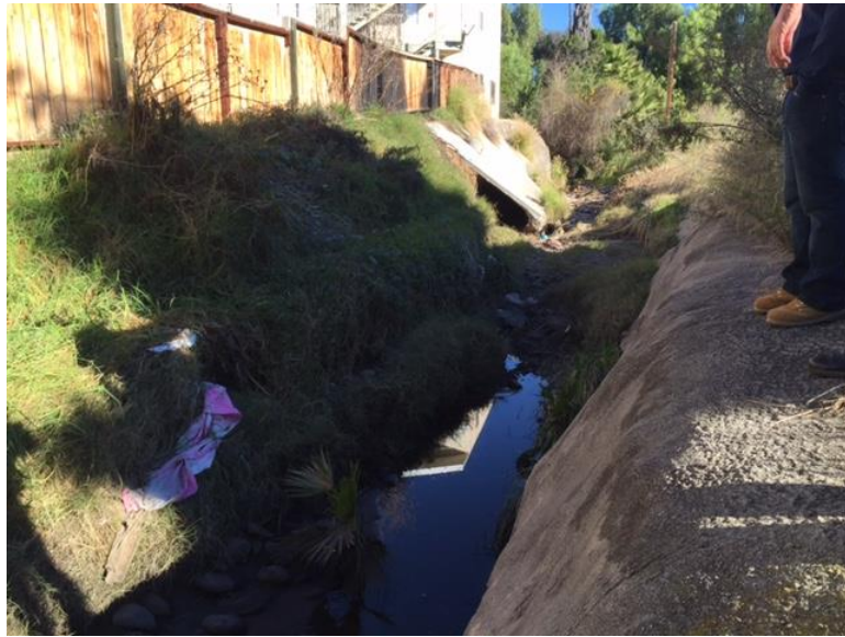
Photograph 3: Looking upstream at sediment and vegetation build up along channel just east of residential parking lot on south end of MMP Map 67; Figure 3a.
