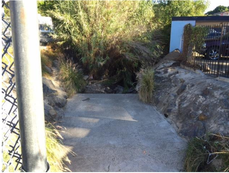
Photograph 11: Looking upstream from the downstream end of Proposed Impact Area Section 2 at sediment and vegetation build up within MMP Map 68; Figure 3b.
