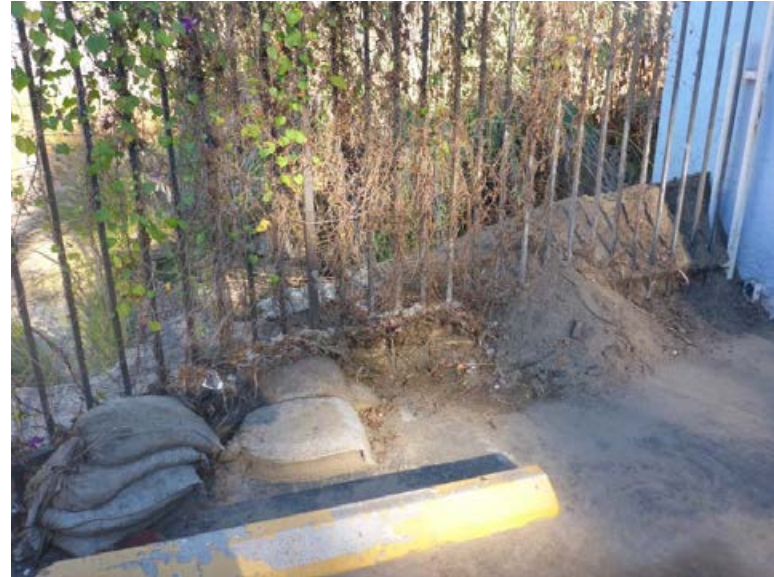
Photograph 10: Evidence of flooding depositing sediment and causing damage to parking structure and lot at 3775 50 th Street property within Proposed Impact Area Section 2 in MMP Map 68; Figure 3b.
