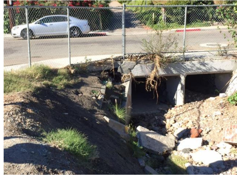
Photograph 15: Evidence of flooding damage to two-box culvert that runs west under Auburn Drive Proposed Impact Area Section 3 in MMP Map 68; Figure 3b.
