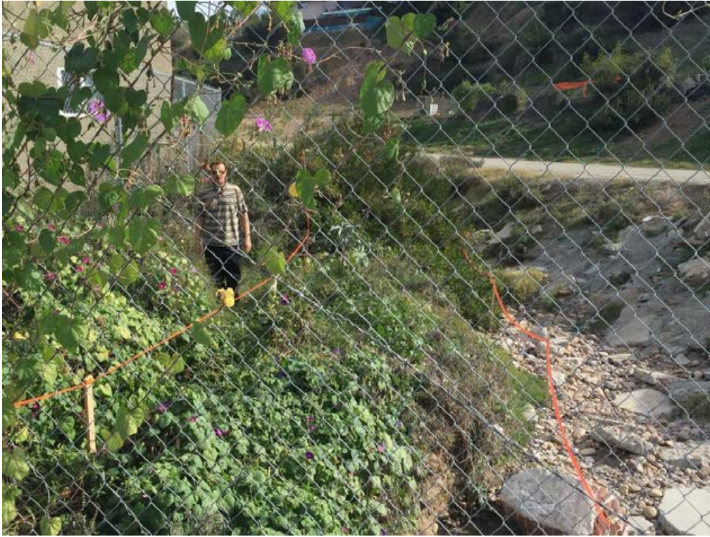
PHOTO 5: Looking upstream (EAST) standing directly above northerly box culvert. Staff is standing at the toe of slope. Removal of sediment will stop outside of the toe of slope and be level with the bottom floor of the channel. Area within orange tape will require the removal of sediment and vegetation.
