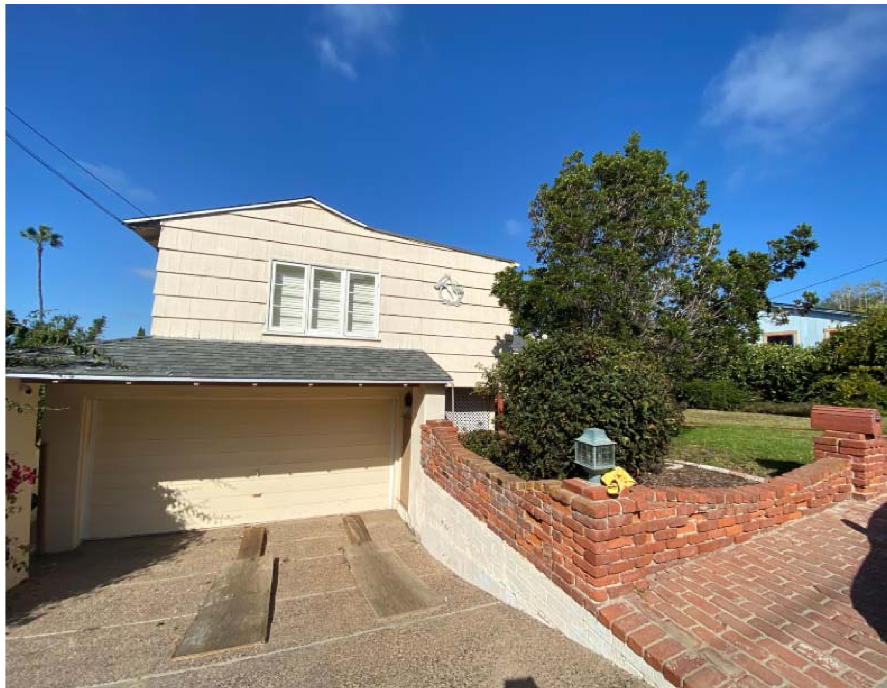
7988 ROSELAND DRIVE SOUTH ELEVATION FROM DRIVEWAY
