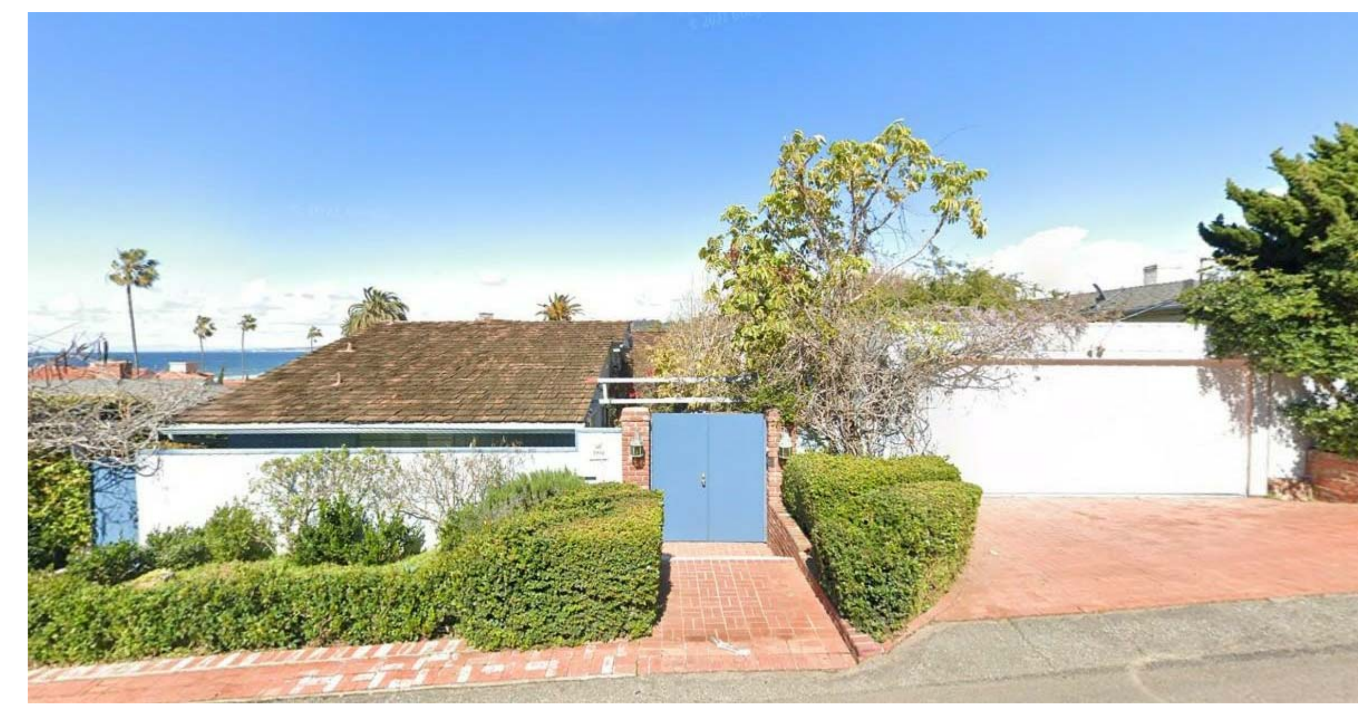
7982 ROSELAND DRIVE SOUTH ELEVATION FROM STREET
