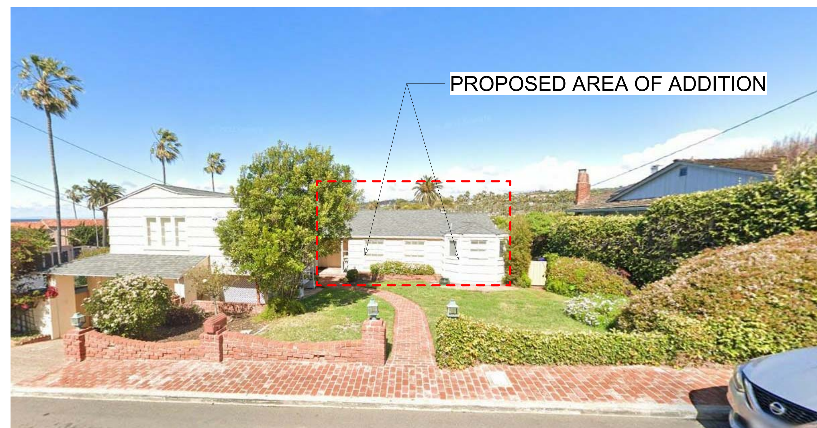
7988 ROSELAND DRIVE SOUTH ELEVATION FROM STREET
