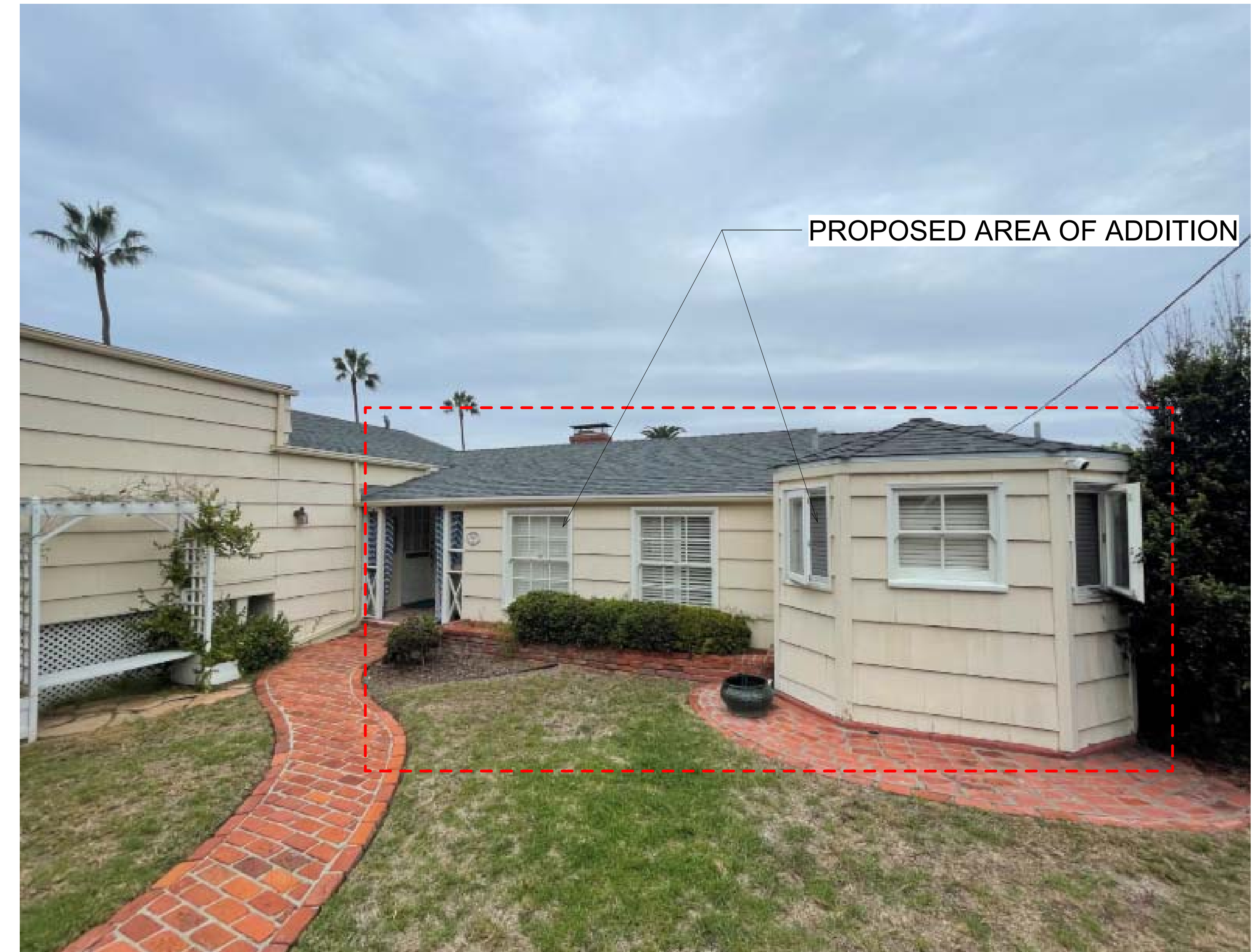
7988 ROSELAND DRIVE SOUTH ELEVATION FROM YARD
