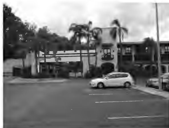
② PARKING LOT LOOKING SOUTH
