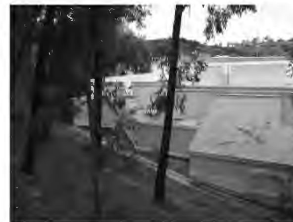
③ SIDE VIEW LOOKING WEST
