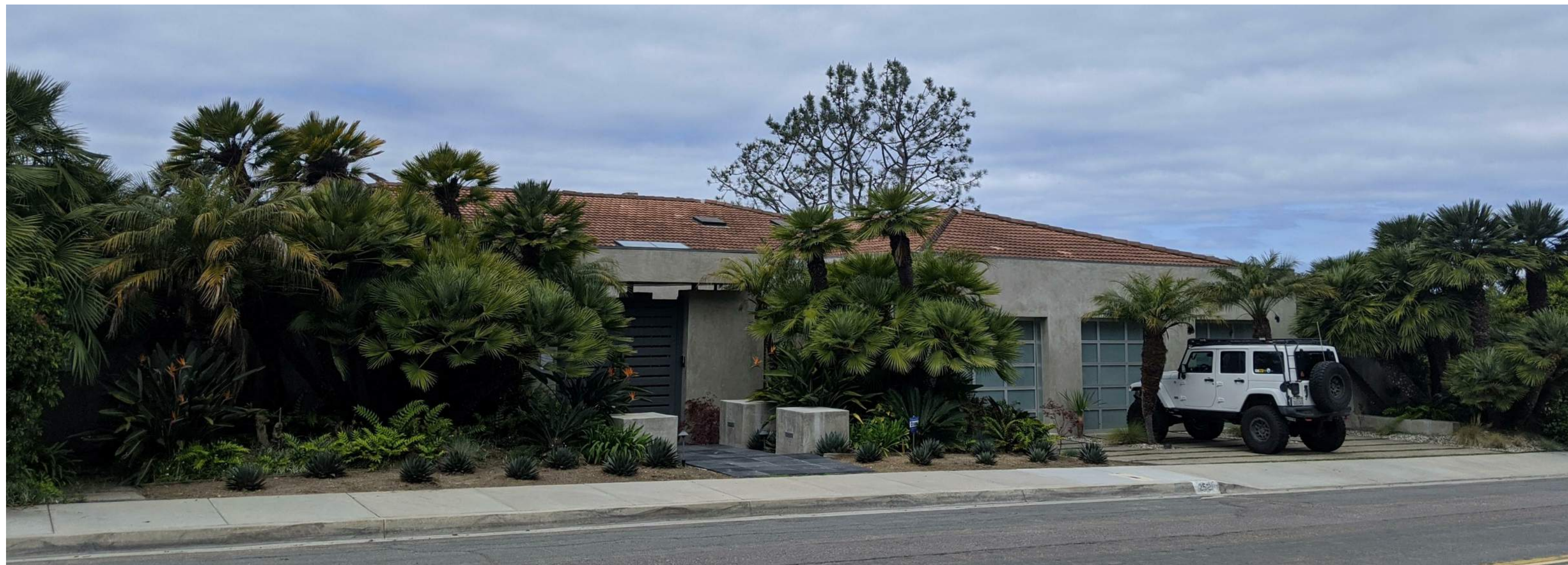
EXISTING ENTRY FACADE
