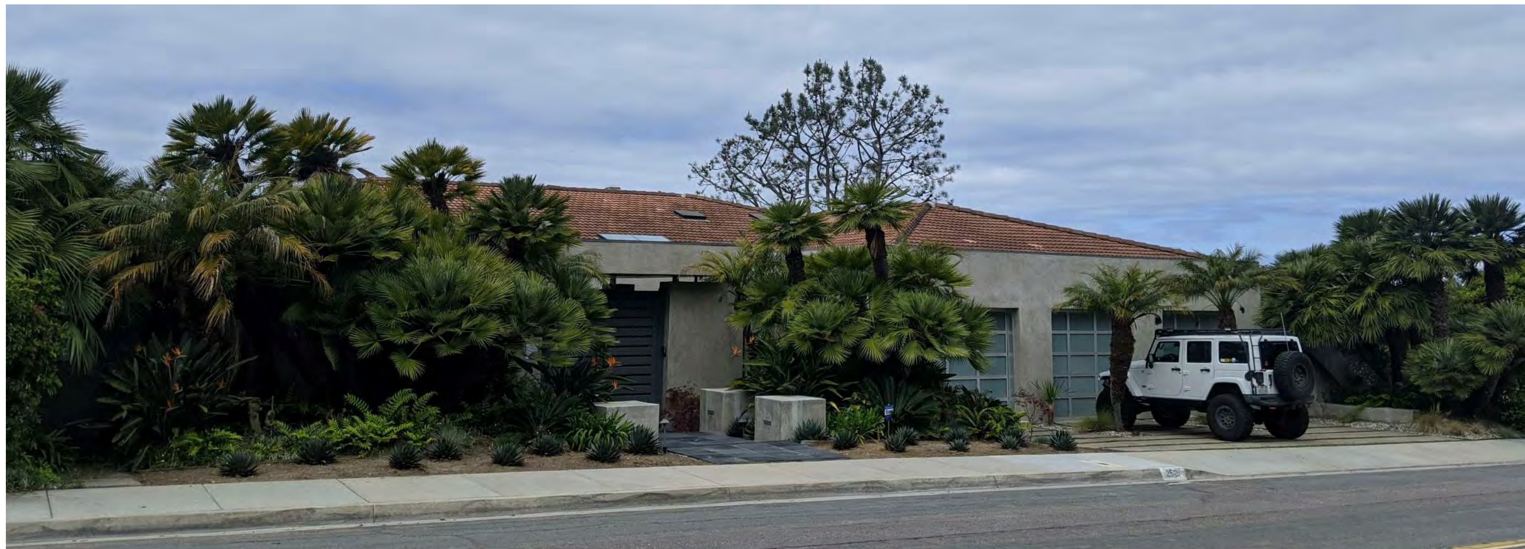
EXISTING ENTRY FACADE
