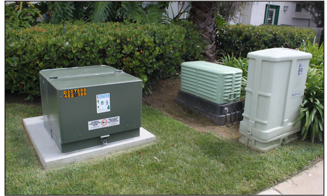
Figure 6: Transformer and cable box
