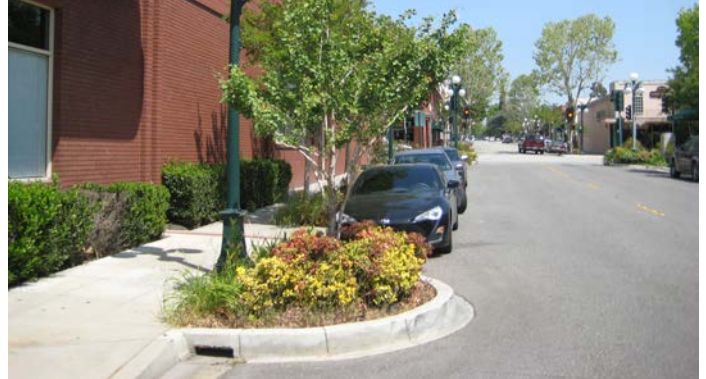
Bulbouts with flow-through planter helps reduce traffic speeds while enhancing the street with landscaping and street trees and stormwater management
