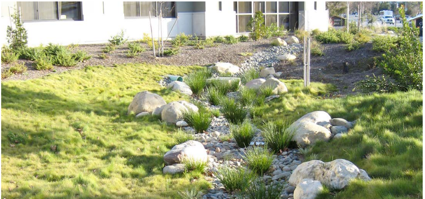
Best Management Practices for new development includes LID techniques to help retain a portion of storm water on-site for infiltration, re-use, or evaporation
