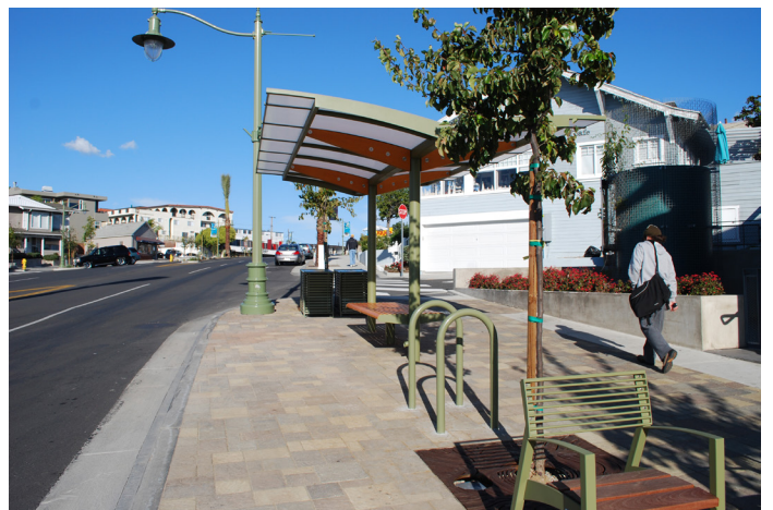
An Enhanced Bus Stop Includes Curb Extensions, Shelter, Bicycle Racks, Seating, Lighting, and Landscaping
