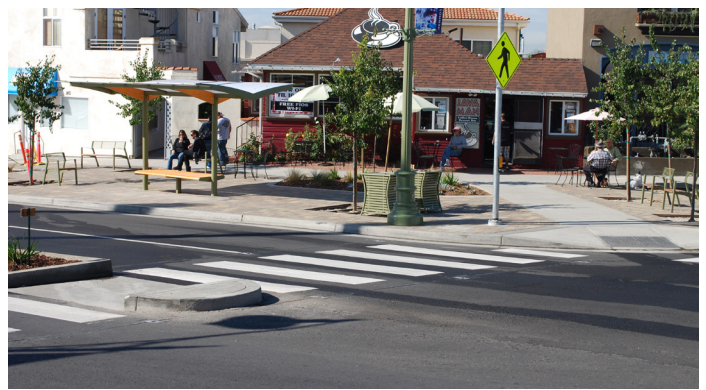
Enhanced crosswalk striping
