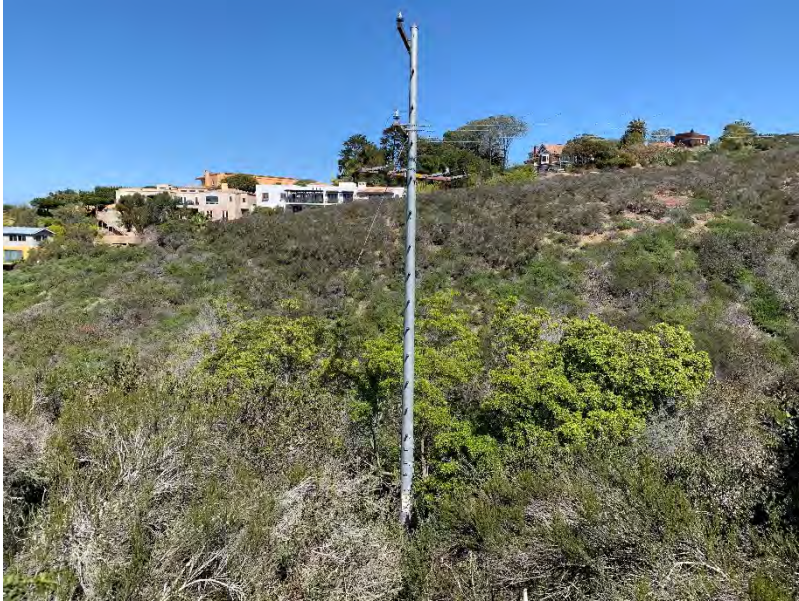
Photo 3. This photo shows the steel pole P836902 located within Southern Maritime Chaparral located in the open space park within the MHPA. This photo will be removed via helicopter with a hand crew that will remove the footings.
