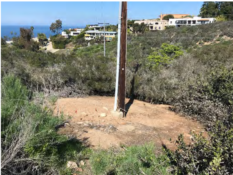
Photo 4. This photo shows P836892 located within Southern Maritime Chaparral located in the open space park in the MHPA. The work area still remains cleared of vegetation from when the pole was replaced in 2016.
