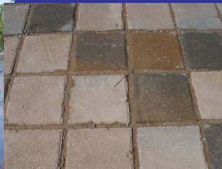
Clogged Permeable Pavement due to "Rogue" Construction
