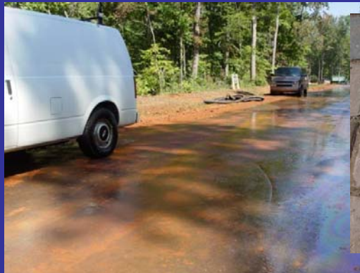
Clogged Permeable Pavement due to "Rogue" Construction
