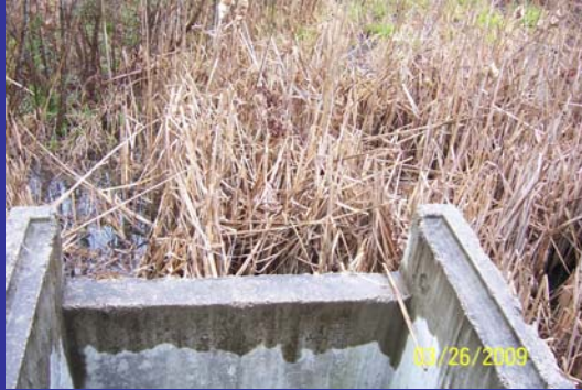
Cattails Clogging Drawdown Structures
