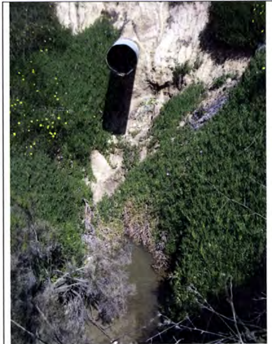
Figure 11. Example of Canyon Area Outfall in Need of Repair
