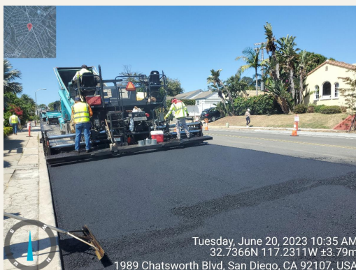
Photos: City crews laying slurry seal in Point Loma.
