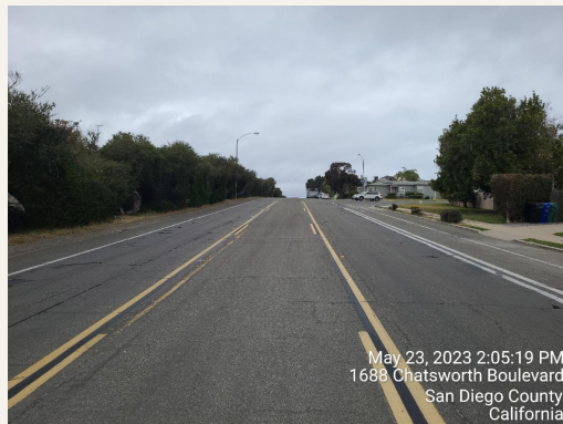
Photos: New slurry seal in Point Loma.
