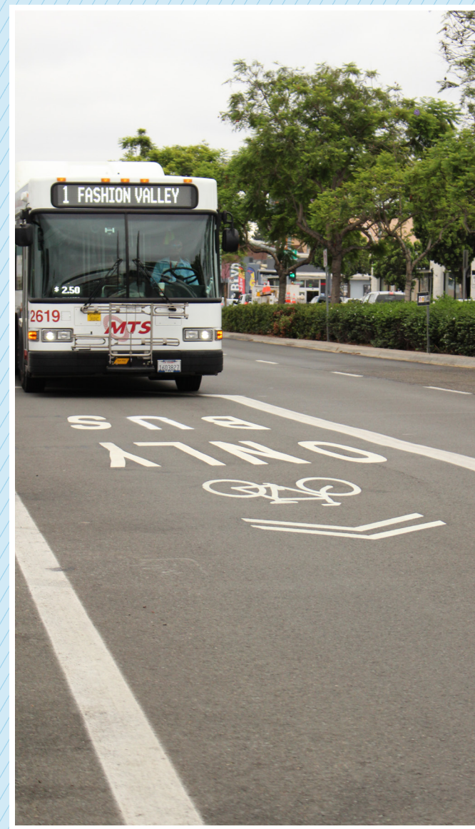
Flexible (flex) lane along El Cajon Boulevard
