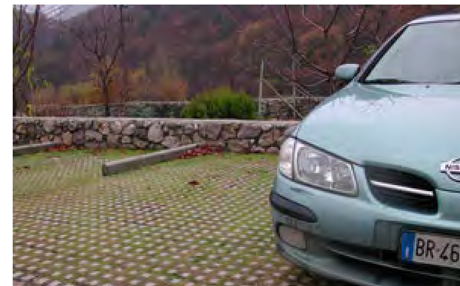
Impermeable (top photo) and pervious (bottom photo) surfaces handle stormwater differently. Pervious surfaces are preferable.
