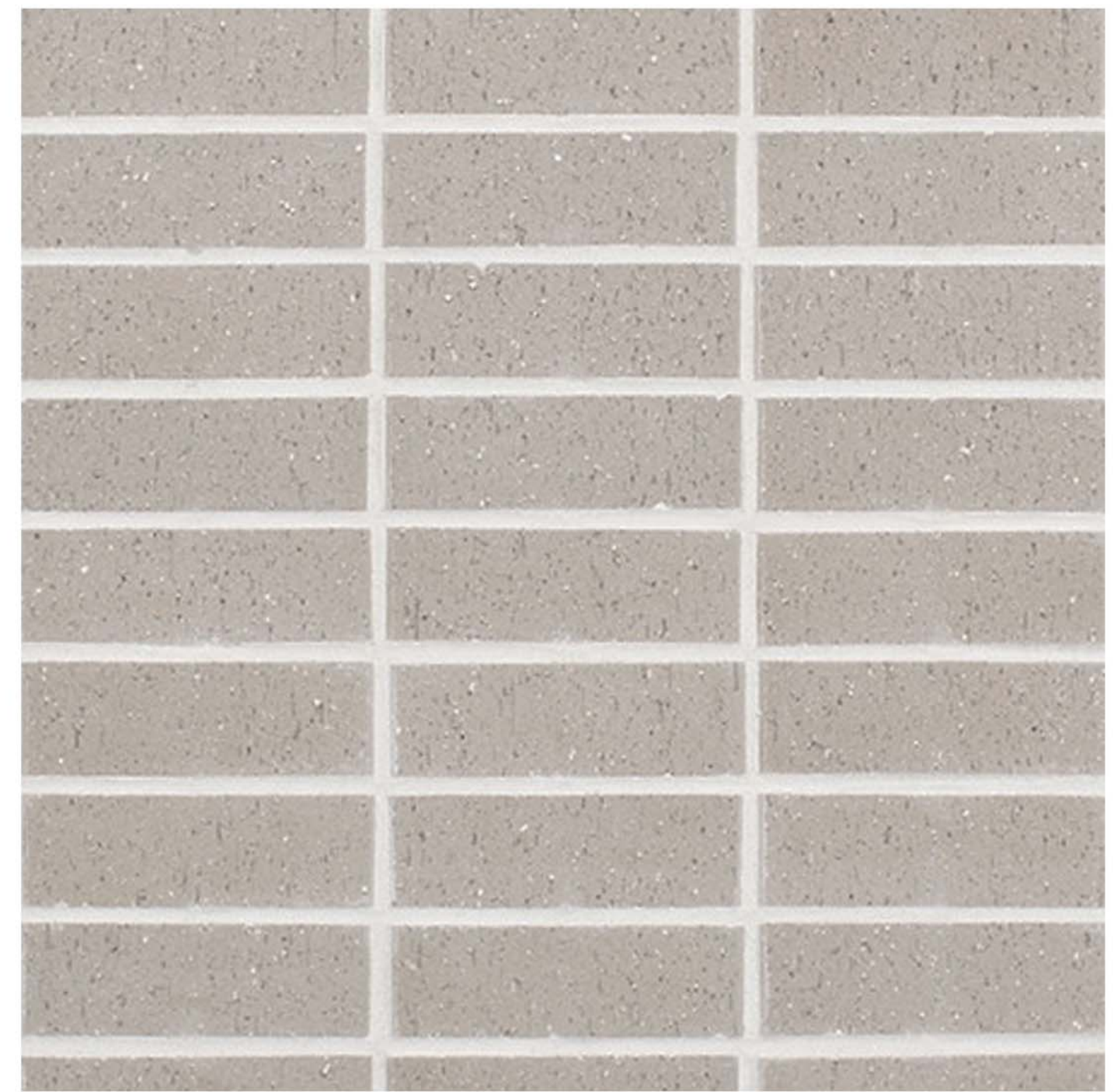
EXTERIOR EXPOSED CMU WALLS
