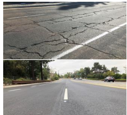
District 5 Roads: Before and After Repaving
