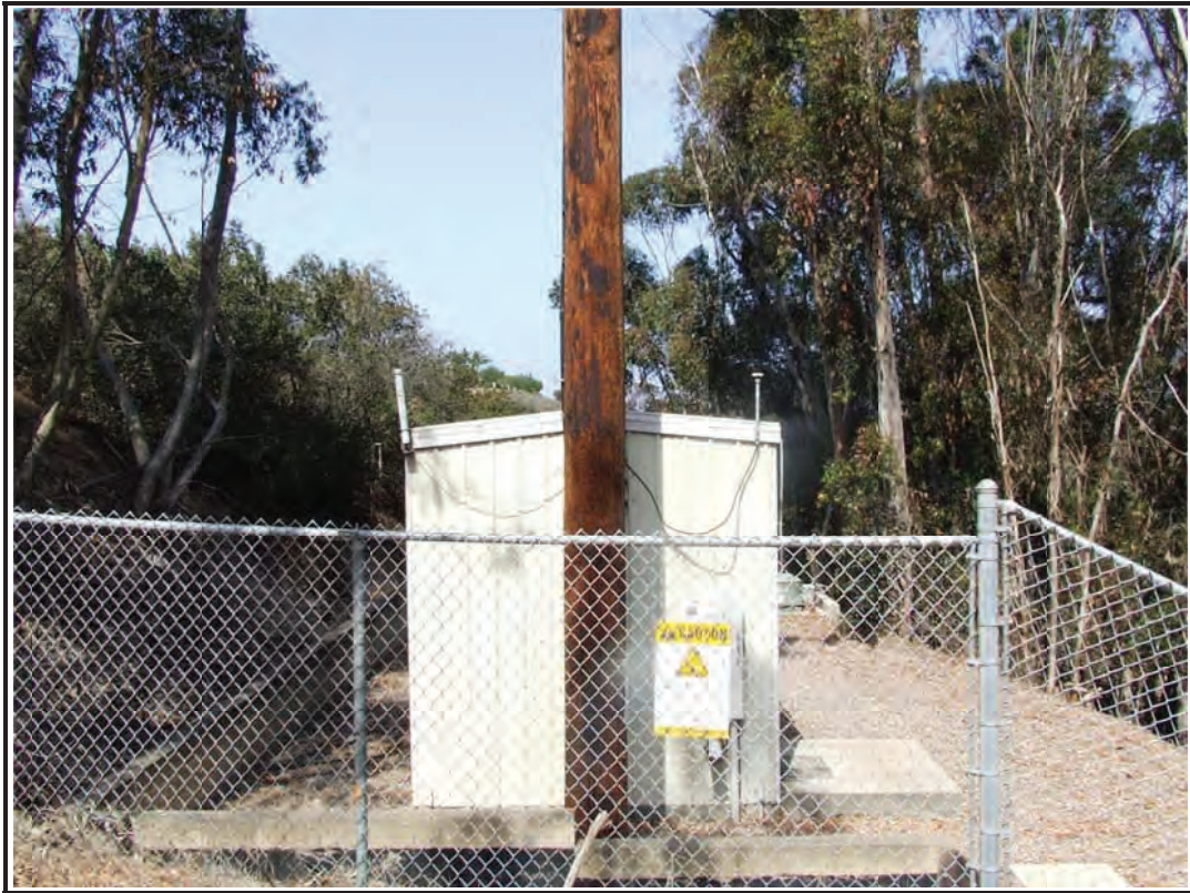
#2 VIEW LOOKING W FROM ADJACENT PROPERTY
