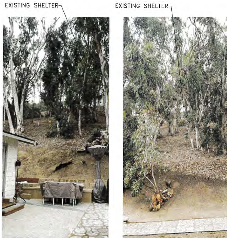
VIEW FROM BOTTOM OF SLOPE TO EXISTING SITE
