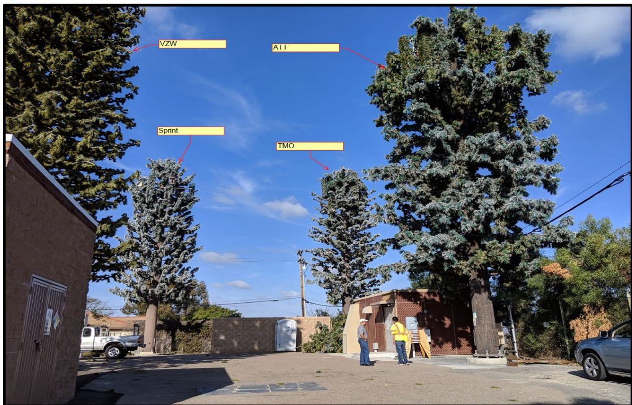
Figure 1: Existing Wireless Communication Facilities on Site
