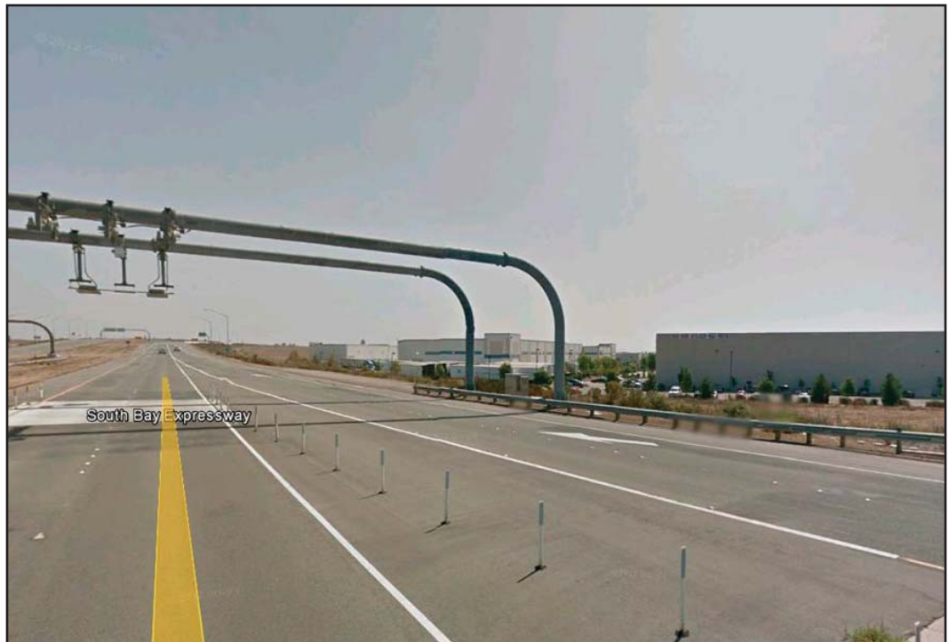
PHOTOGRAPH 10: On SR-125 East of Aviator Road Looking South
