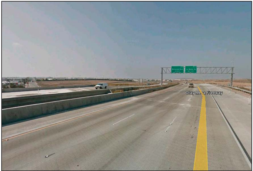
PHOTOGRAPH 9: On SR-905 at Airway Road Overpass Looking North
