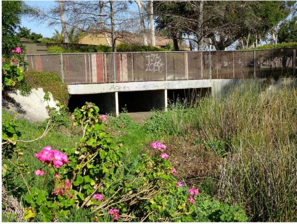
Figure 13. Box Culverts at Lower End of Reach 3
