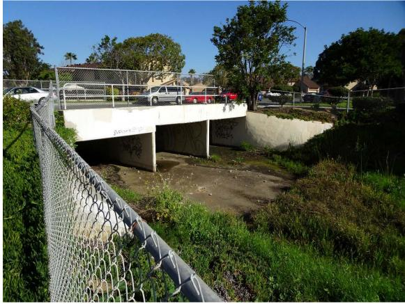
Figure 9. Box Culverts at Cerrissa Court (Grade Control between Reach 2 and 3)
