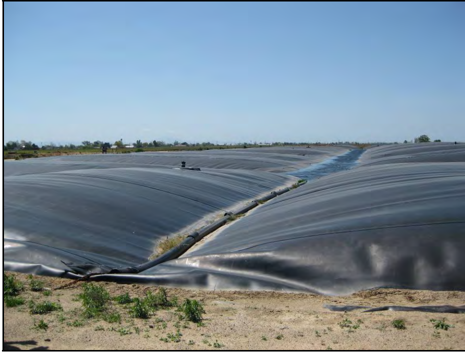
Figure 11-3 Covered Lagoon Digester
