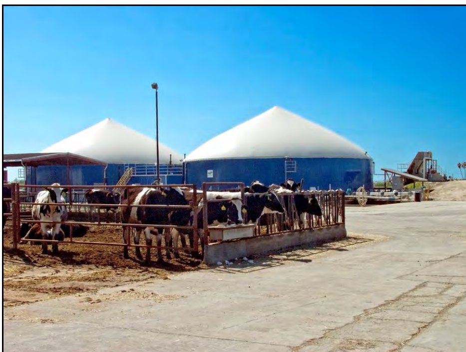
Figure 11-2 Complete Mix Digester Tanks
