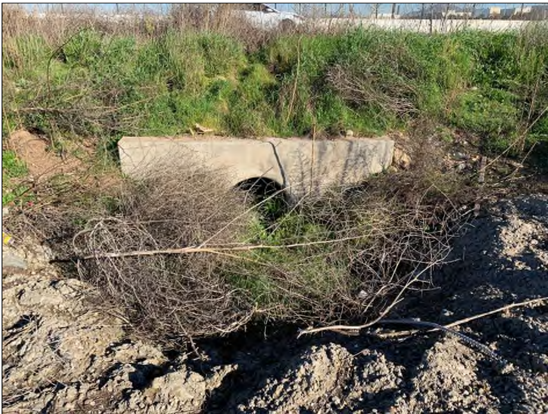
Photograph No. 8 Drainage headwall along north-central perimeter of the Site.
