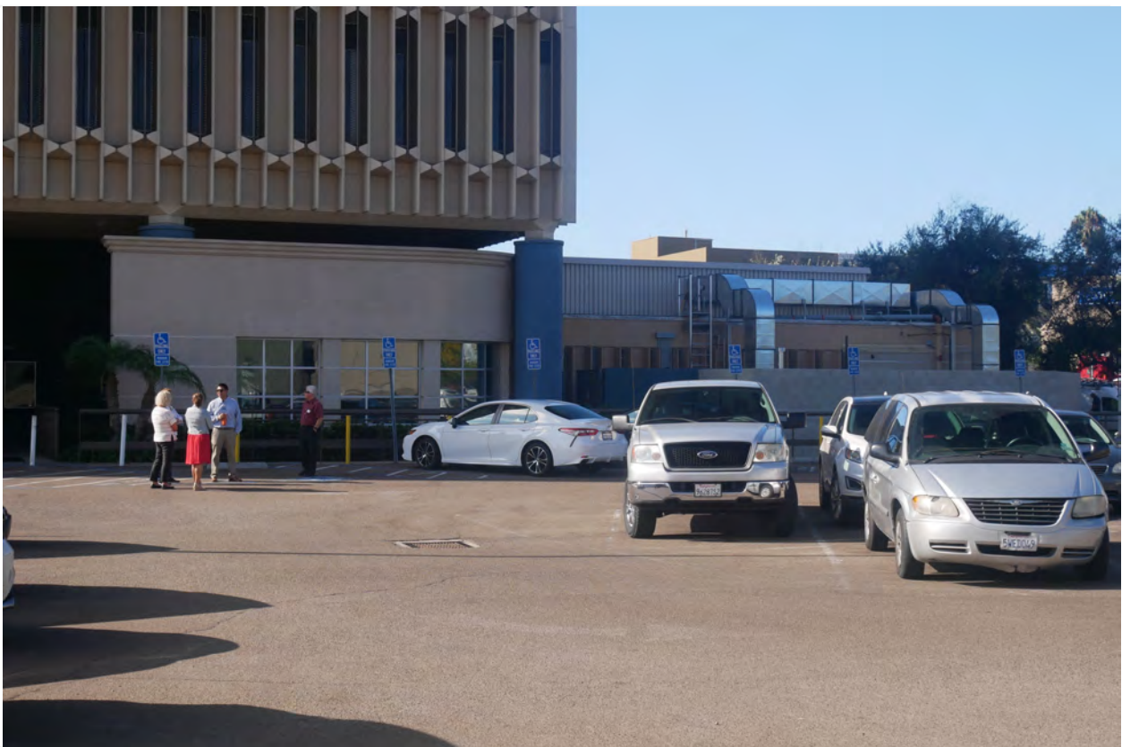
Photograph #24: North elevation, one-story west wing covered with mechanical equipment and lobby and original columns are enclosed with stucco.
