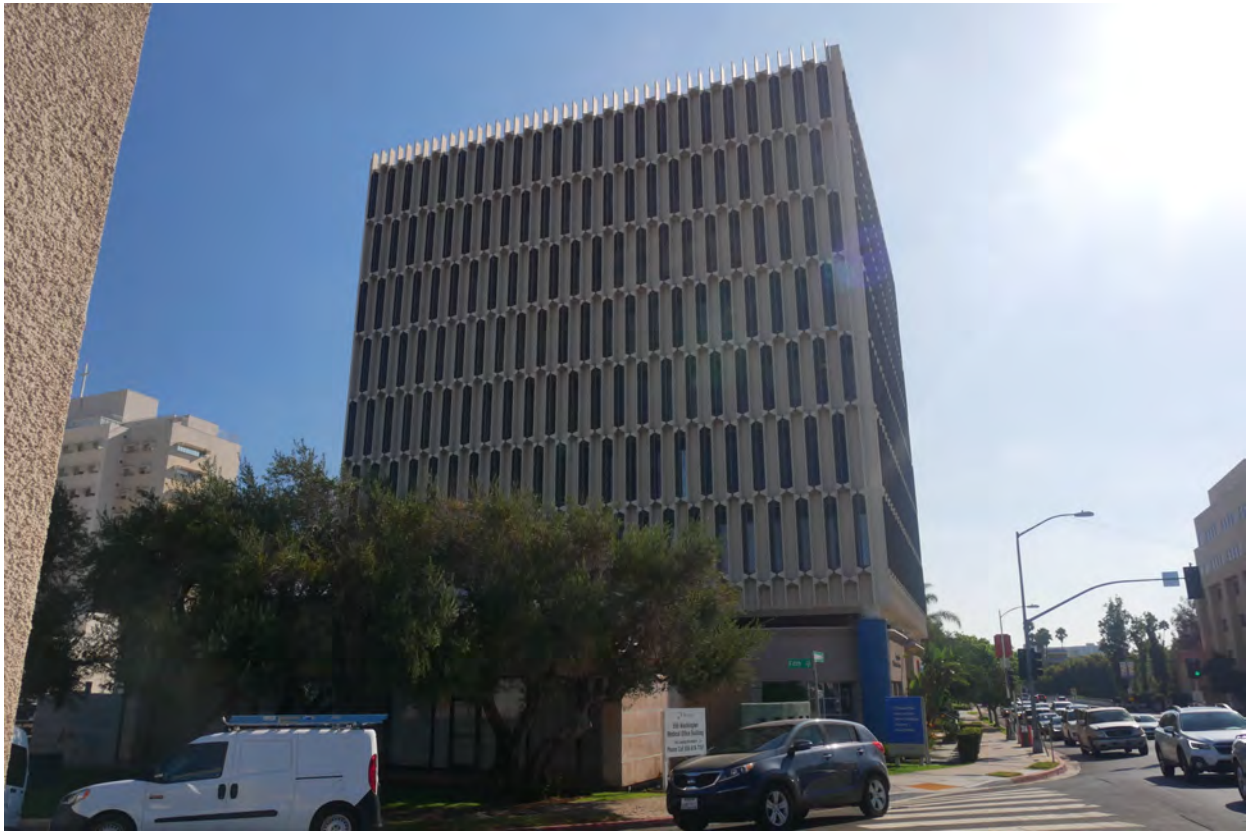
Photograph #21: West elevation.
