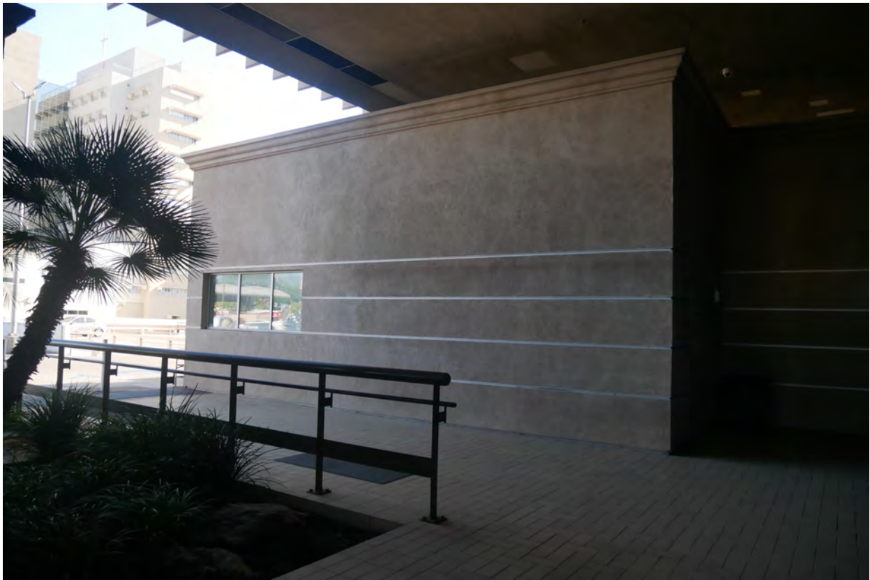
Photograph #32: Formerly open-air lobby, now enclosed with full height walls and additional enclosed space under tower. Enclosed space is out-patient surgical center.
