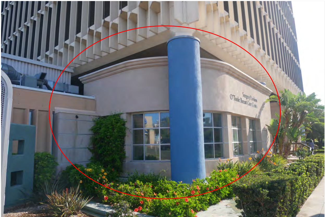
Photograph #19: Front, lobby enclosure and column addition, all new in 2003.
