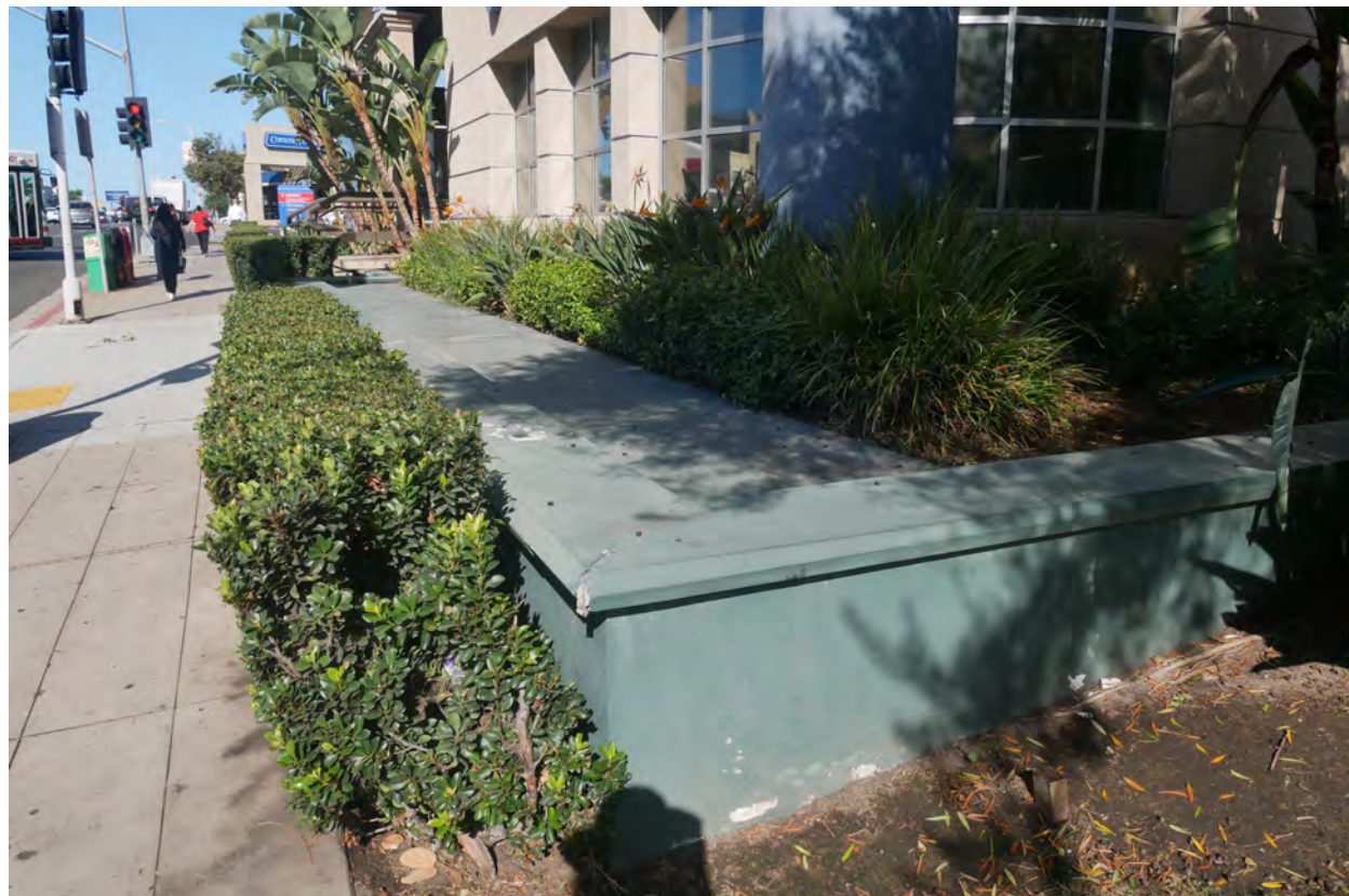
Photograph #18: South elevation, planter wall and lobby enclosure.
