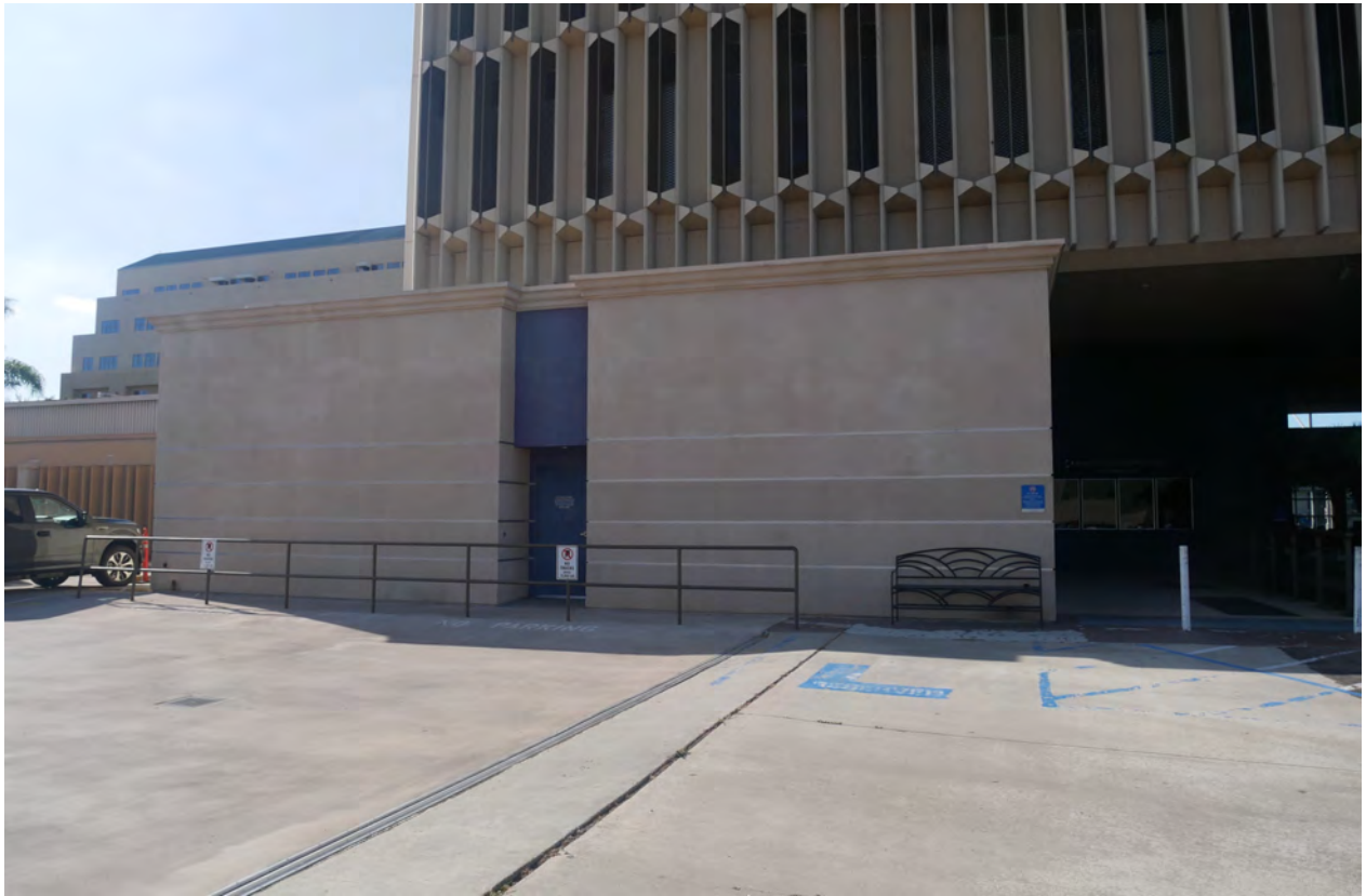
Photograph #26: Rear, north elevation. Out-patient surgical pavilion.
