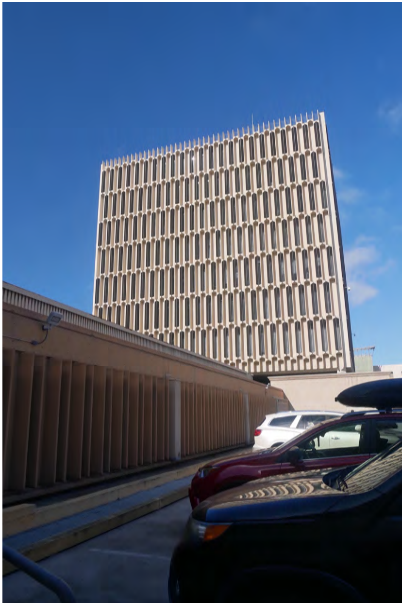
Photograph #28: East elevation of tower and north elevation of one-story wing (east side of parcel) with stucco and mechanical additions.
