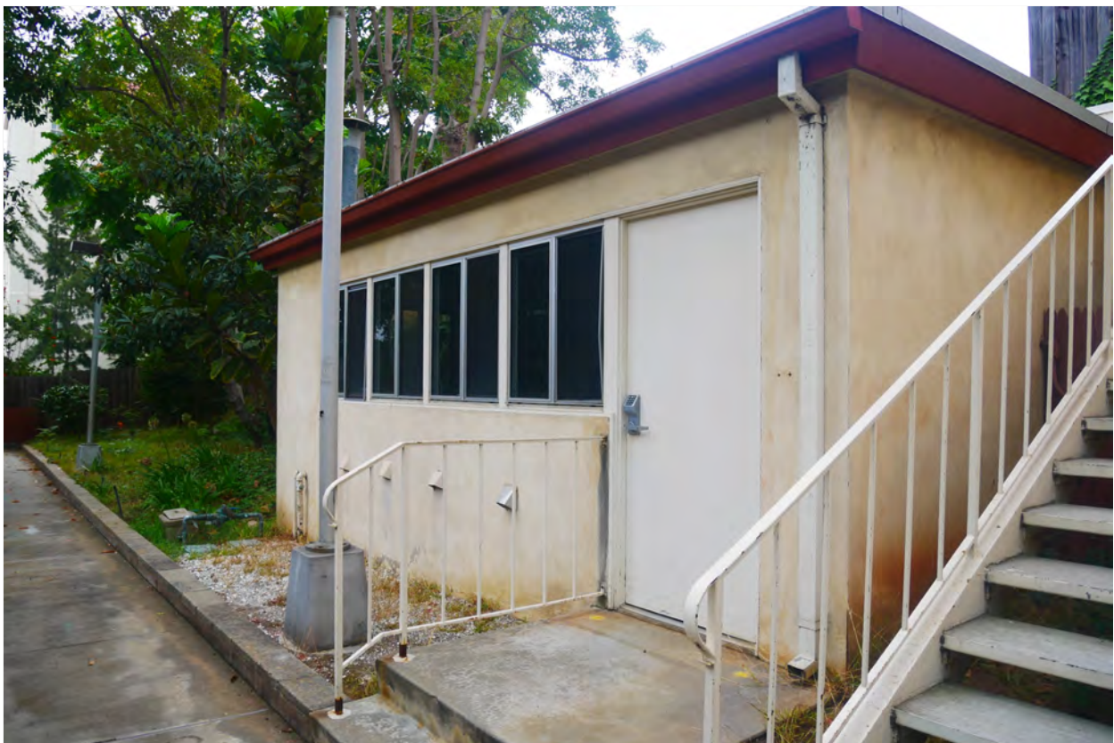
Image #55: Mercy Manor laundry building
