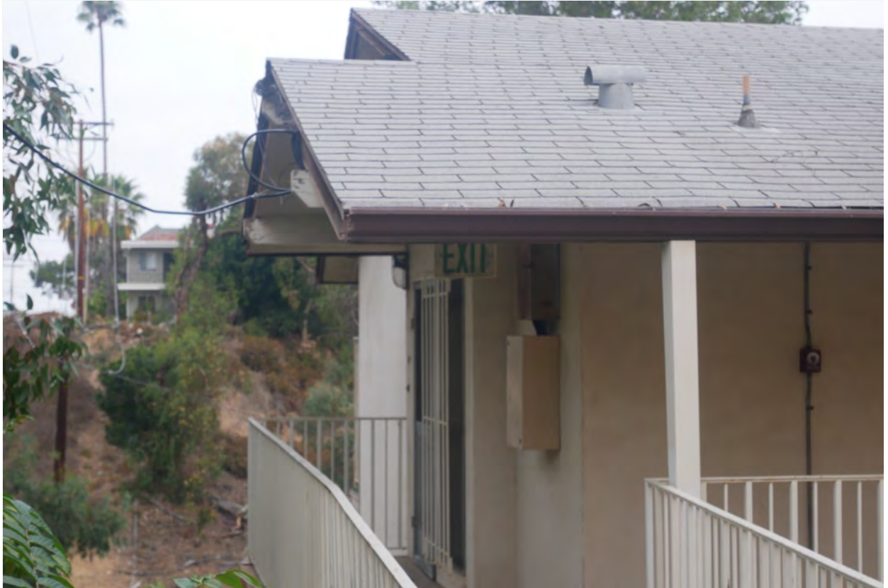
Image #52: Mercy Manor third floor, southwest elevation
