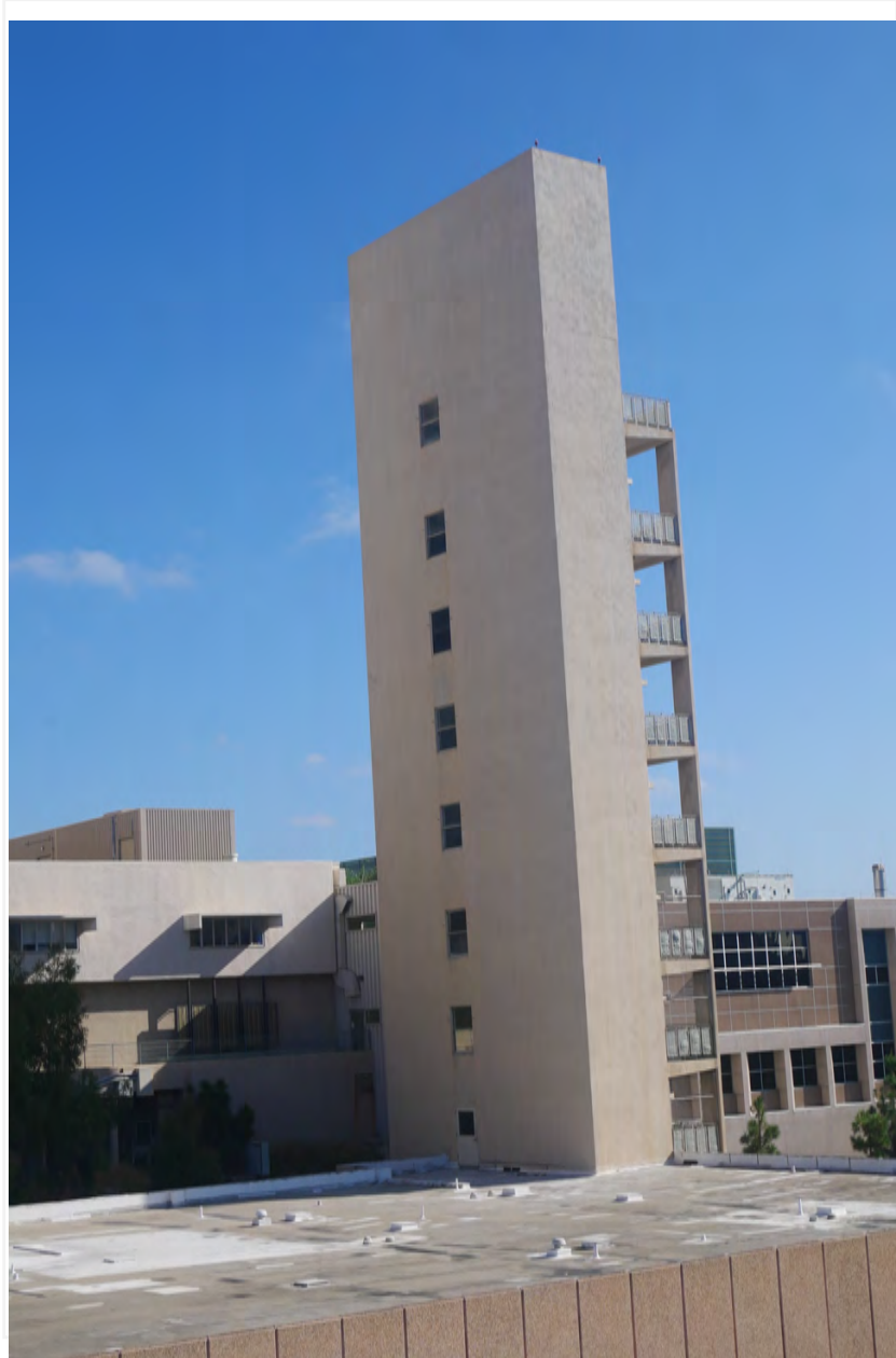
Image #48: Mercy Behavioral Health, elevator and stair tower, south elevation
