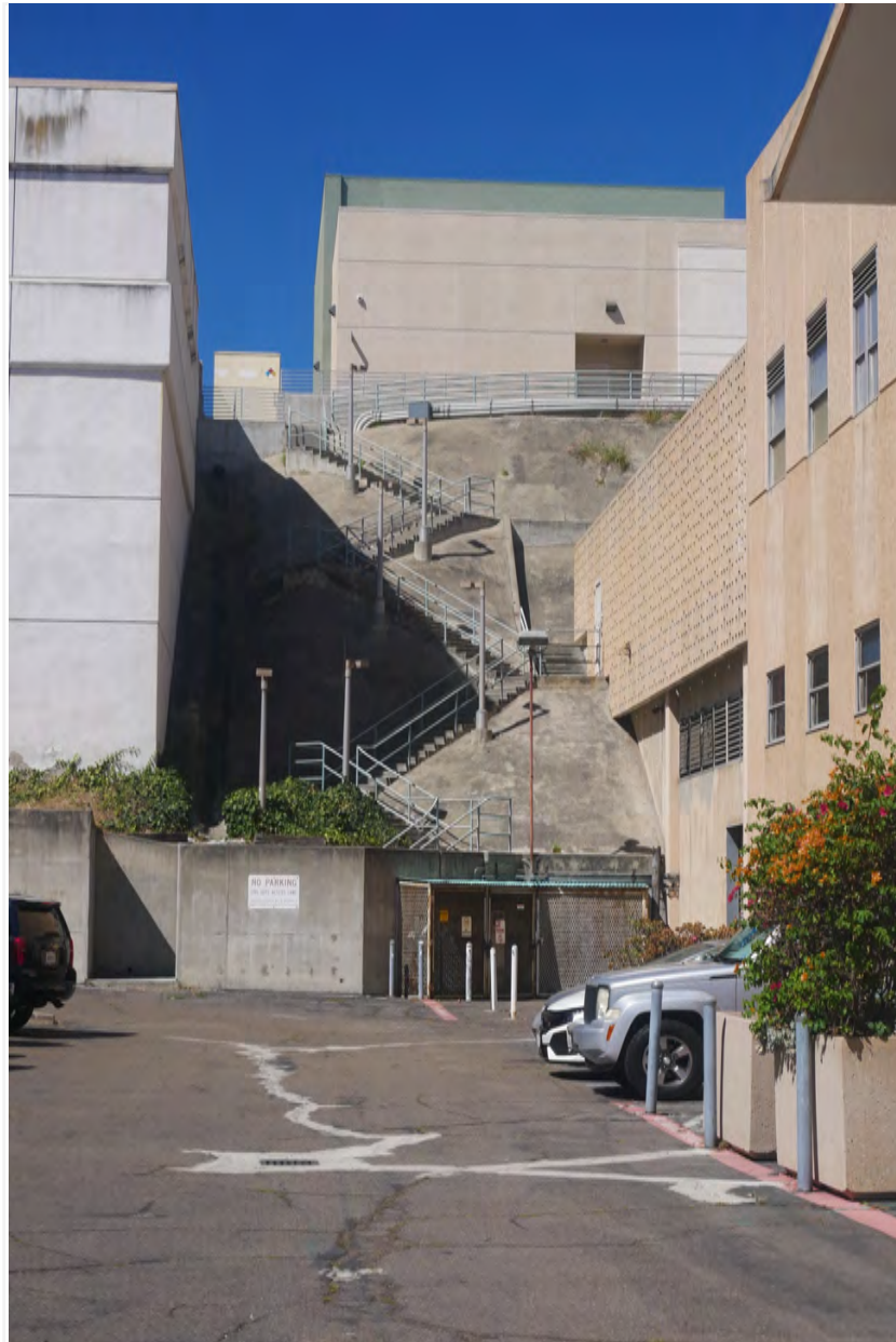
Image #41: Mercy Behavioral Health, retaining wall
