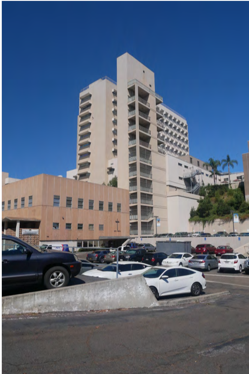
Image #49: Mercy Behavioral Health, elevator and stair tower, southeast elevation
