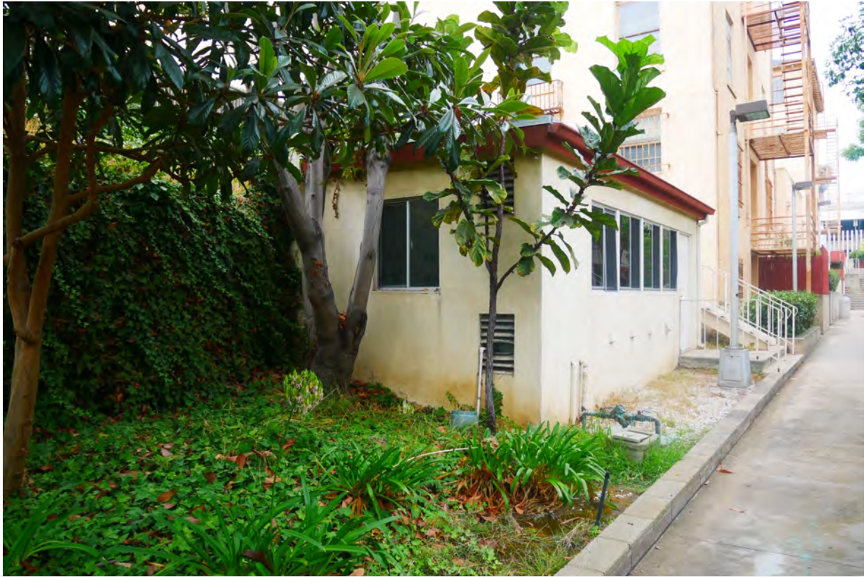
Image #54: Mercy Manor laundry building
