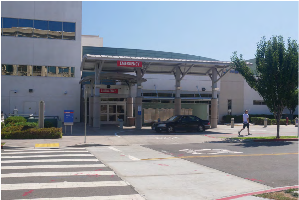
Image #30: Scripps Mercy Hospital, front, east elevation (2012 Emergency Department)
