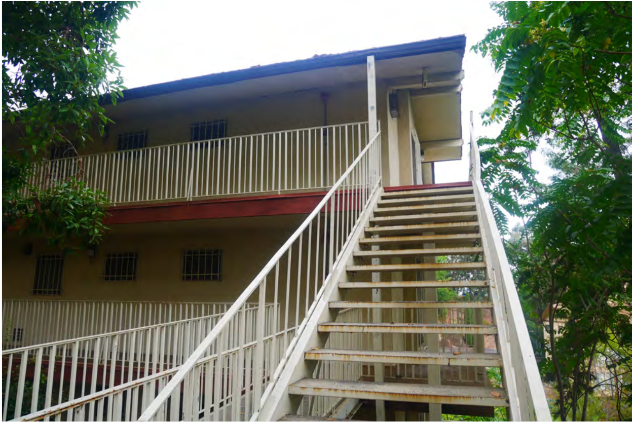
Image #56: Mercy Manor south east end of building
