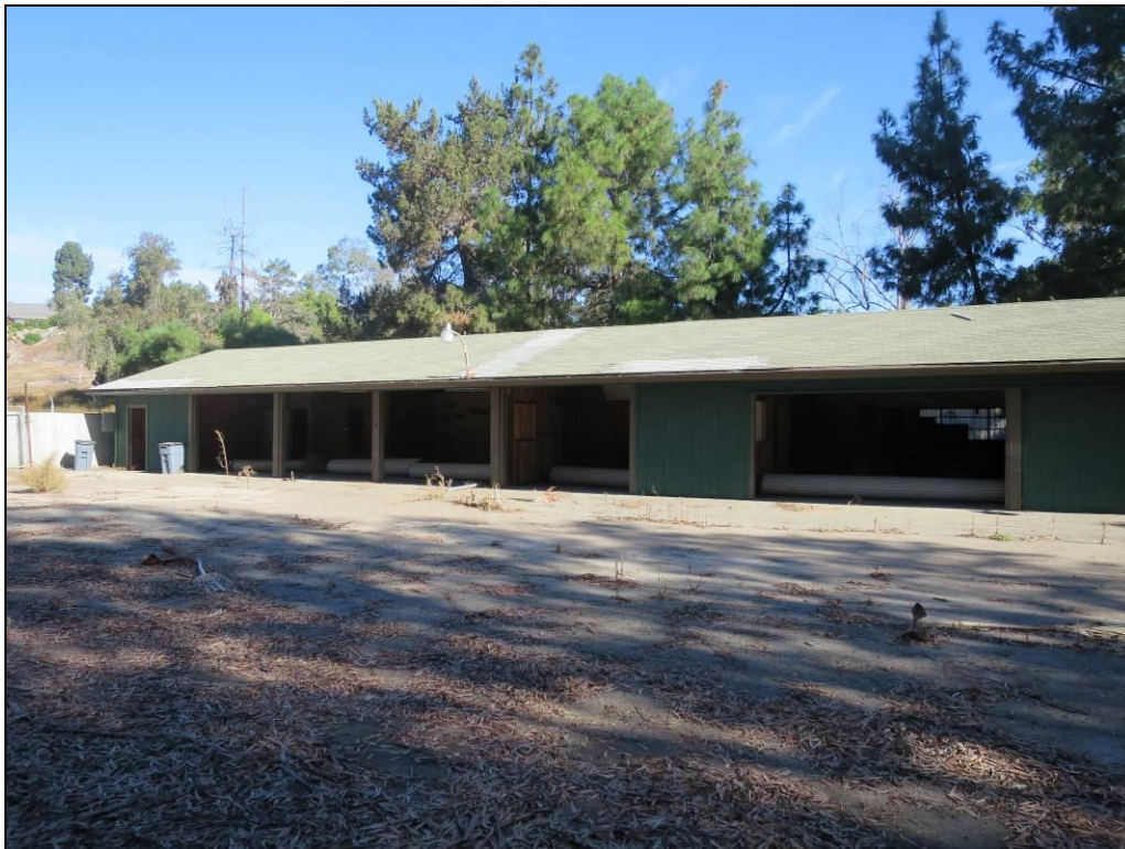
Figure 3: Southwest elevation of structure facing northeast. (photograph by IS Architecture 2017)
