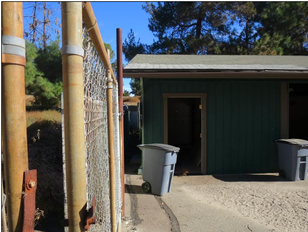
Figure 5: Northwest elevation of structure facing northeast. (photograph by IS Architecture 2017)
