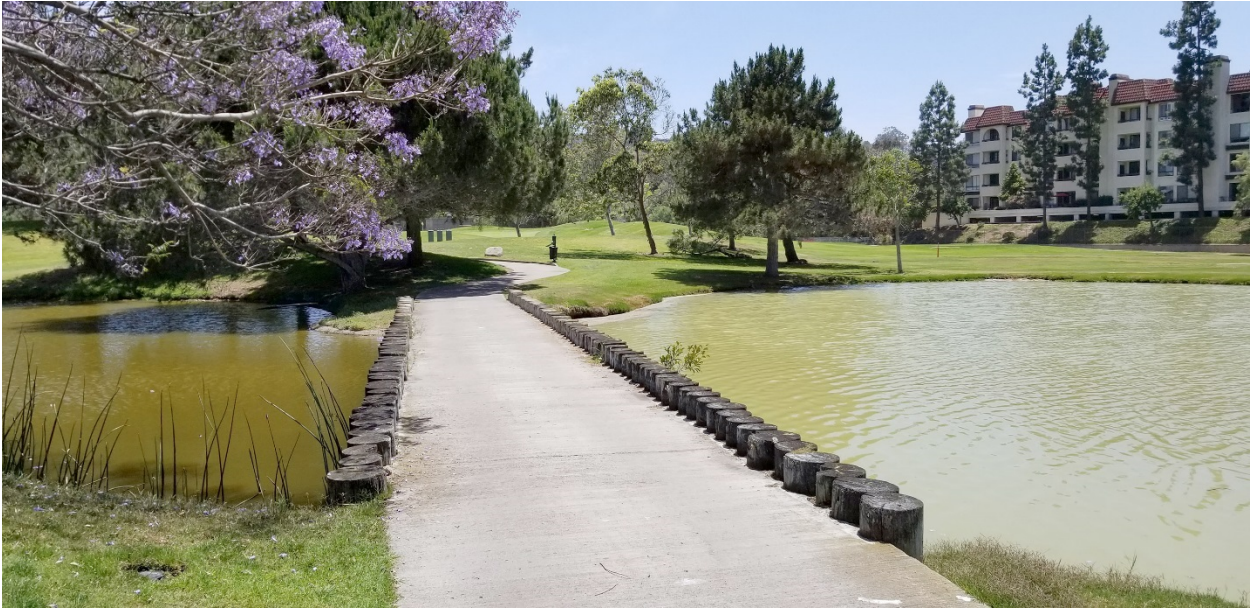
Figure 71. An example of a concrete golf cart foot bridge on the fourth hole of the Friars course. Photograph taken facing southwest.
