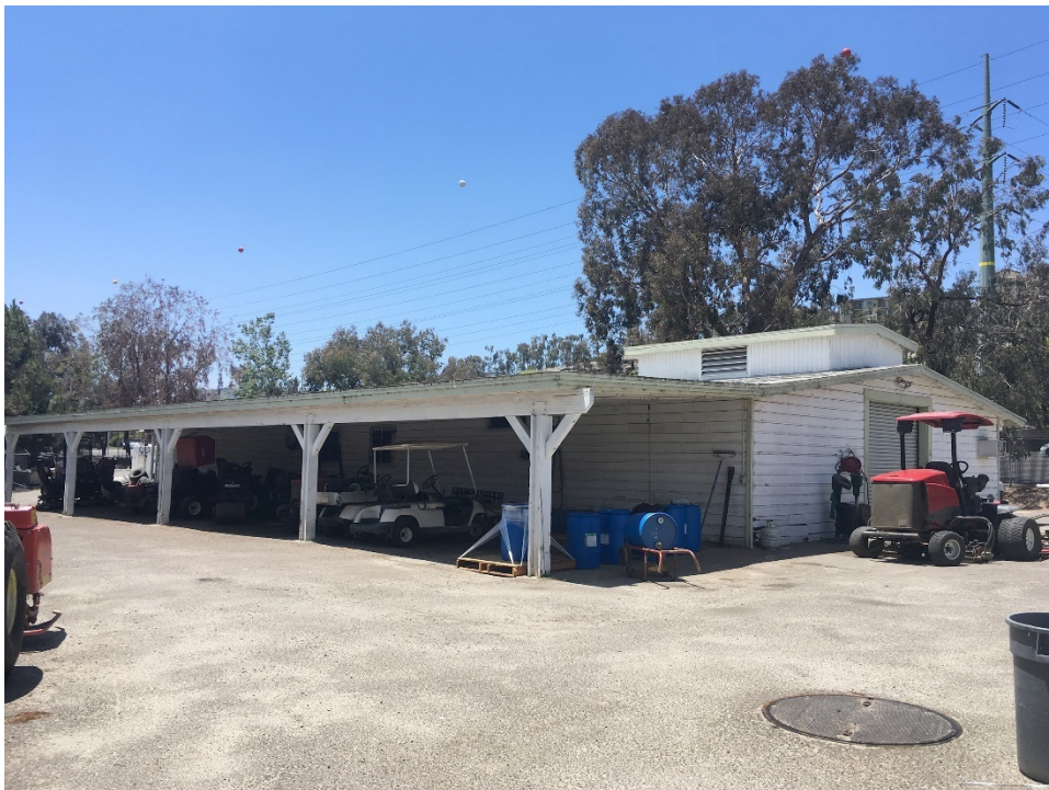
Figure 63. The west shed, showing the shelter spanning the south façade and the clerestory section. Photograph taken facing northwest.
