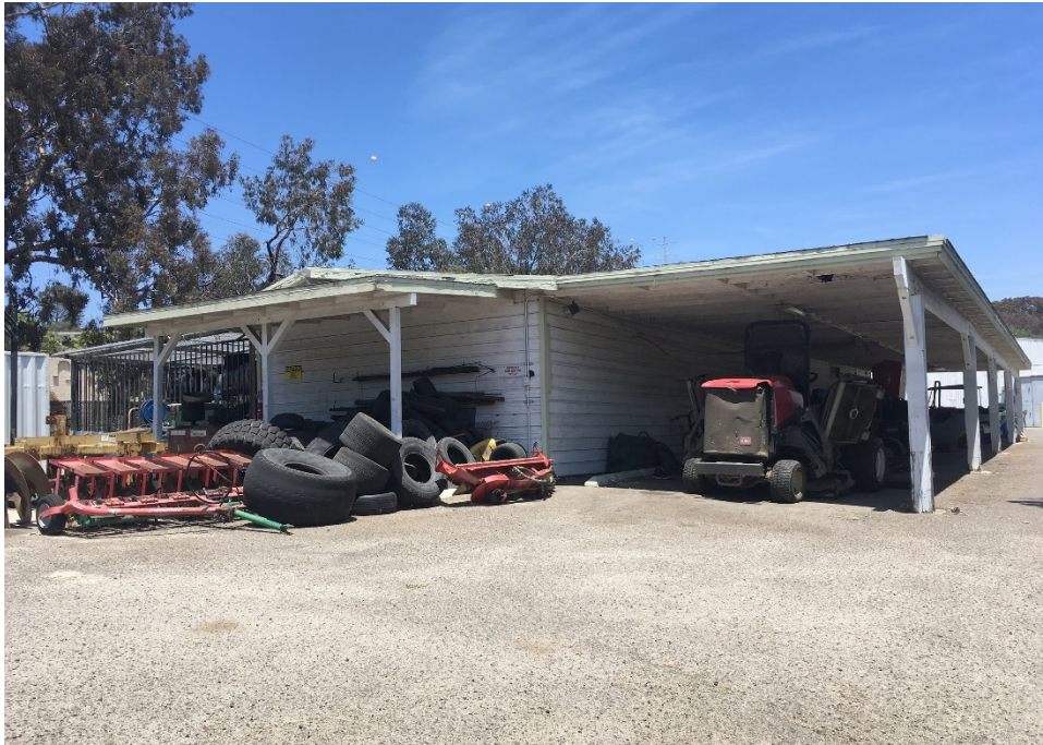
Figure 62. The west shed, showing two attached shelters. Photograph taken facing northeast.
