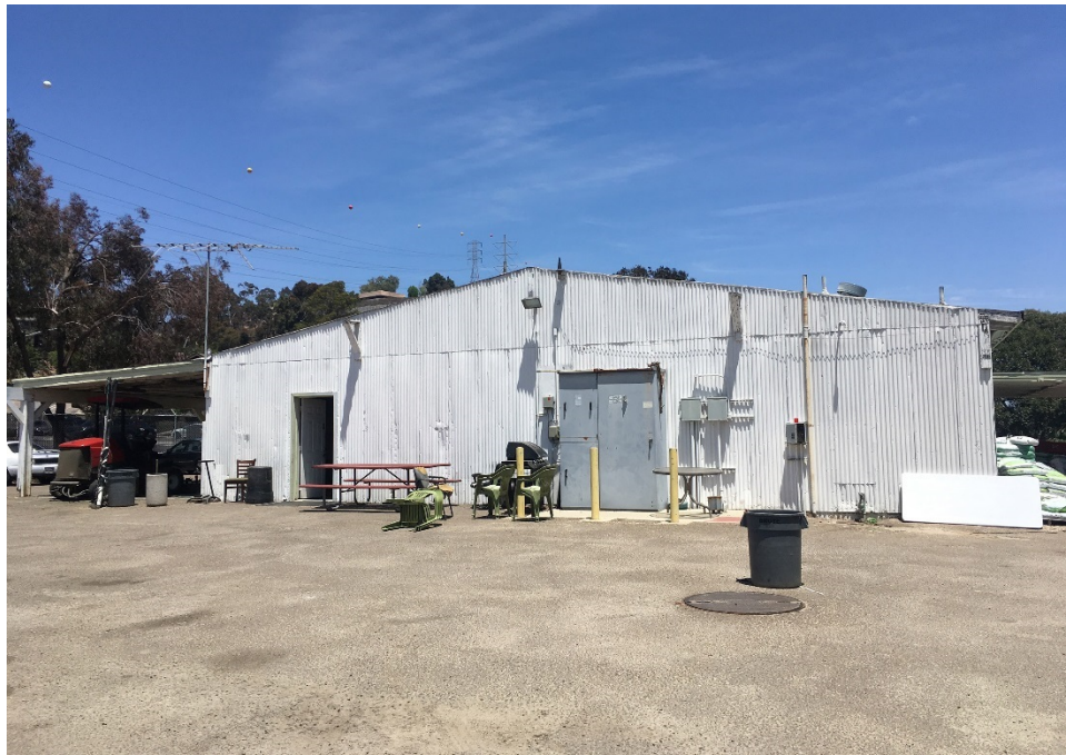
Figure 66. The east shed, showing the west facade. Photograph taken facing east.
