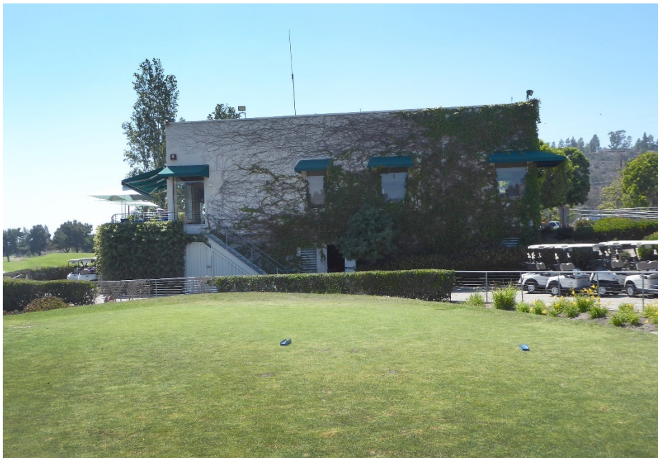
Figure 61. Clubhouse. Photograph taken facing northwest.
