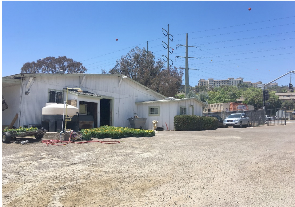
Figure 64. The east shed, showing the gable-roofed wing. Photograph taken facing northwest.
