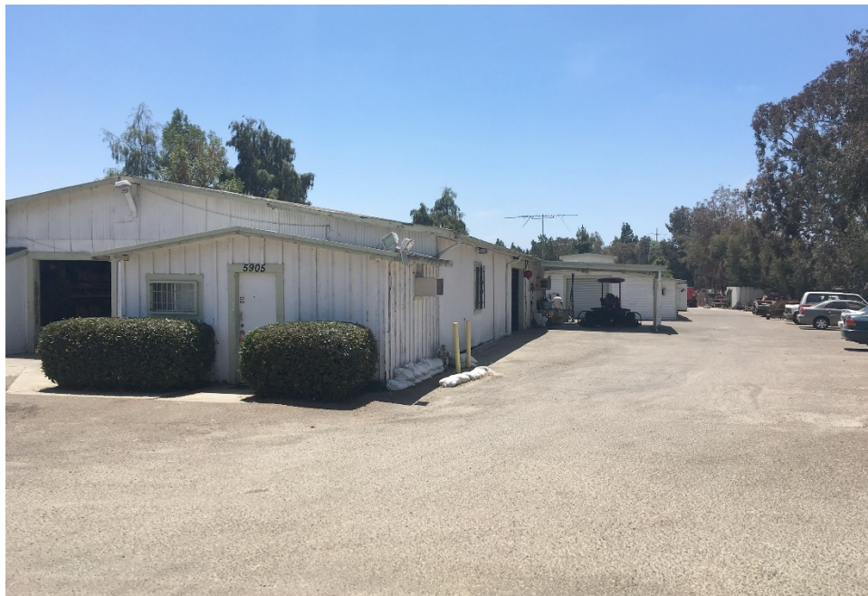
Figure 65. The east shed. Photograph taken facing southwest.
