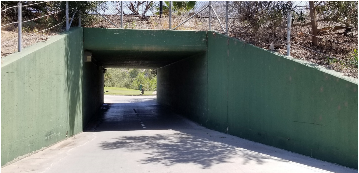
Figure 72. Tunnel located at the end of Presidio 9. Photograph taken facing north.
