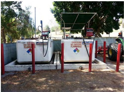
**Photo 12**: View of 1,000 gallon diesel and gasoline ASTs in secondary containment in the maintenance area in the central portion of the Site.
