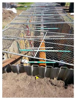
**Photo 7**: View of the SDGE 17" gas line in the central portion of the Site.
