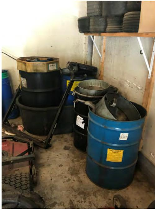
**Photo #29** View of waste oil, waste antifreeze, waste oil filters, and waste absorbent drums located within the maintenance building. The waste oil and waste anti-freeze drums are located within a secondary containment unit, while the waste oil filters and waste absorbent drums are stored on bare flooring.
