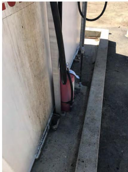
**Photo #18** View of gasoline and diesel AST secondary containment. Minor staining observed on the concrete secondary containment.
