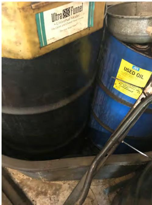
**Photo #30** View inside secondary containment unit for the drums. Free liquid was observed in the bottom on the secondary containment unit.
