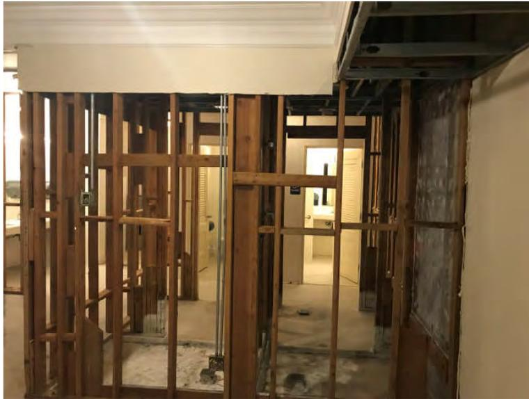
**Photo #5** View of remodeling area in the restroom and locker room area of the clubhouse. The remodeling is a result of water flooding damage.
