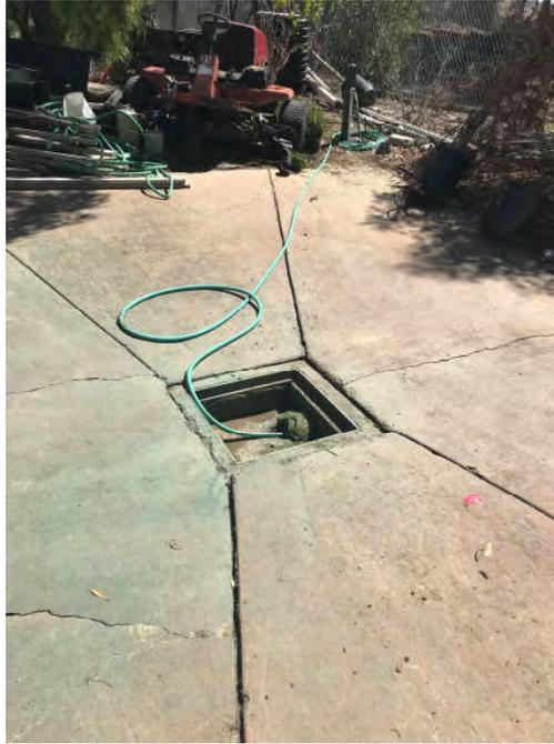
**Photo #37** View of drain located southeast of the maintenance building. Green staining was visible on the concrete surrounding this drain.
