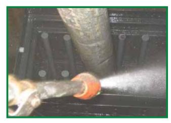
Spray Down and Clean Cartridge Filter Housing
