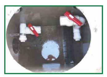
Open Discharge Chamber Lid to Asses Wetland Media Flow Rate and Replace Drain Down Filter Near Bottom
