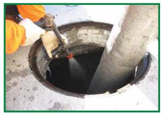
Vacuum out the Sediment Chamber
