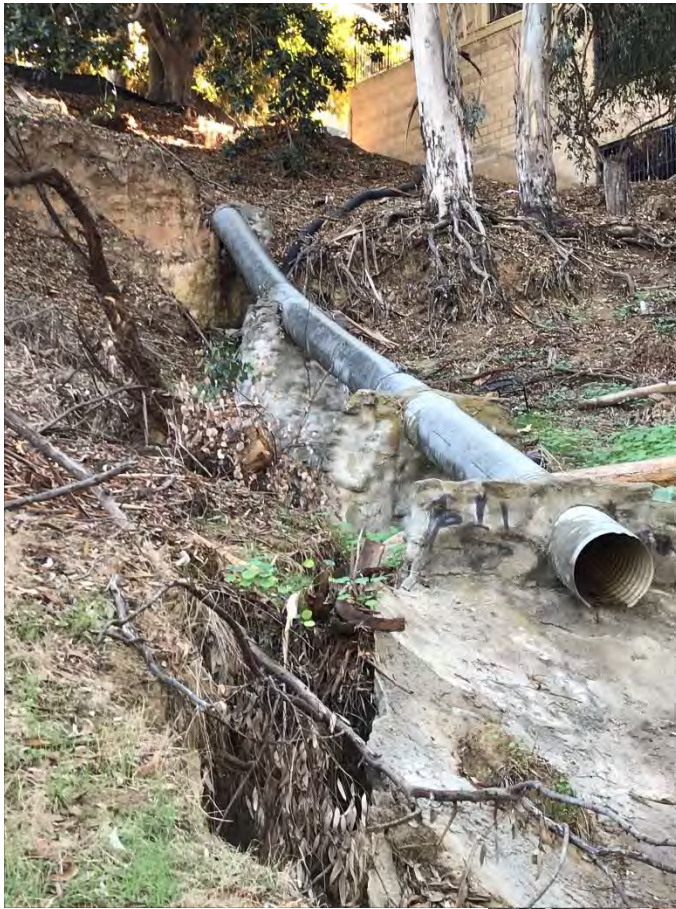
Photo 3.1: Close up of outfall of a CMP that is likely from street SD inlet above. Note erosion below where pipe emerges from bank indicating it is broken. As a result, most of the water bypasses the end of the pipe and the concrete that has been poured to carry the water. Cut-off walls have kept the pipe in place, but the pipe is compromised.
