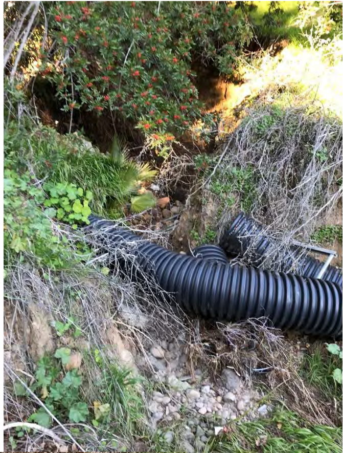
Photo 1.5: Chaotic flow and storm drain debris below the broken pipe.
