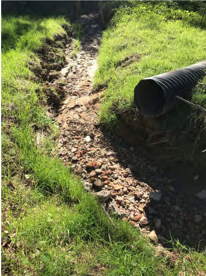
Photo 1.18: A CMP, presumably from an SD placed to put water into the creek downstream of the trail crossing. The CMP is titled up so that water does not flow freely.
