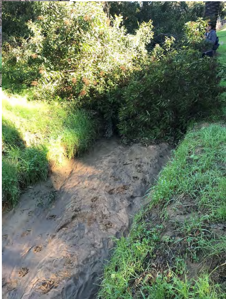
Photo 1.27: A laurel sumac has fallen over into the channel in where the bank has been eroded at the start of the final reach.
