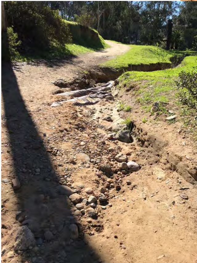
Photo 1.17: Looking south where Drainage 1 crosses the trail. The ends of two CMPs are visible but where they start is unknown. The drainage quickly reforms a bed and bank after crossing the trail.
