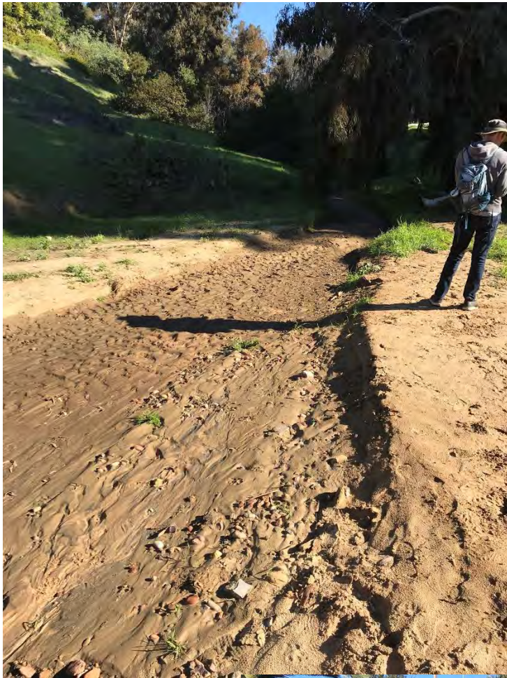
Photo 1.28: Drainage 1 enters the filled detention basin with banks of less than 1 foot.
