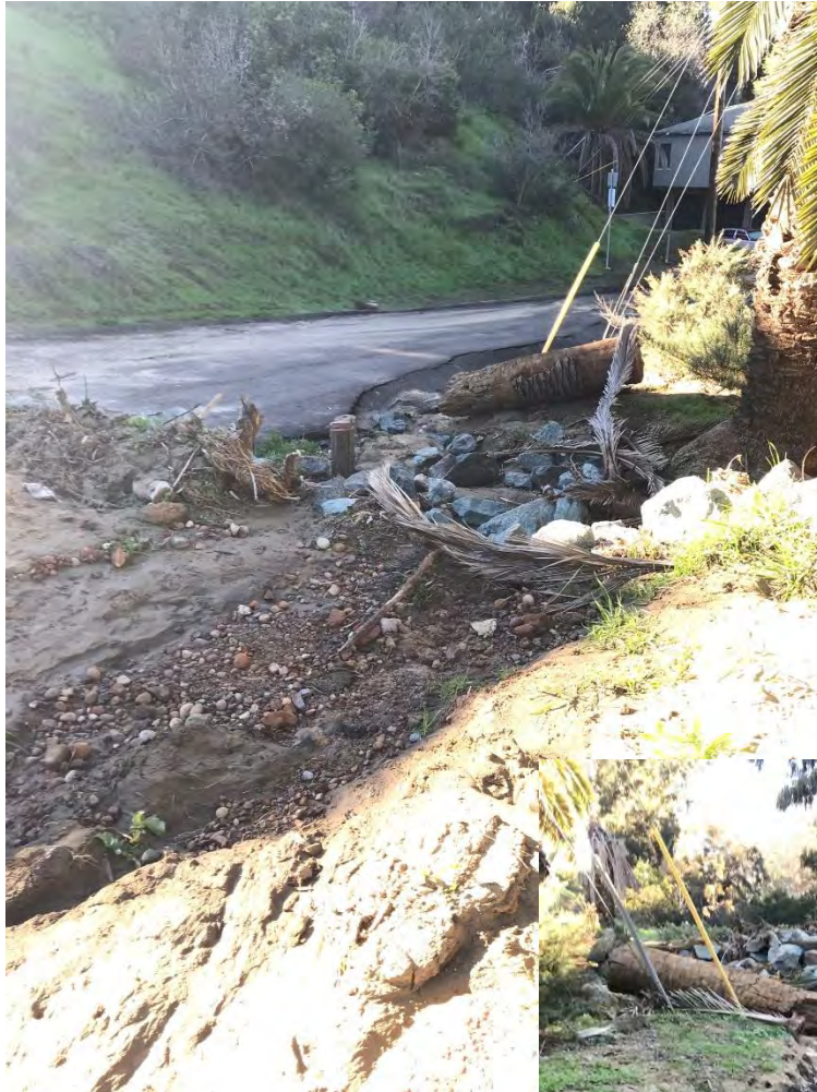
Photo 1.30: at the western end of the detention basin the water has overtopped and undermined the riprap.
