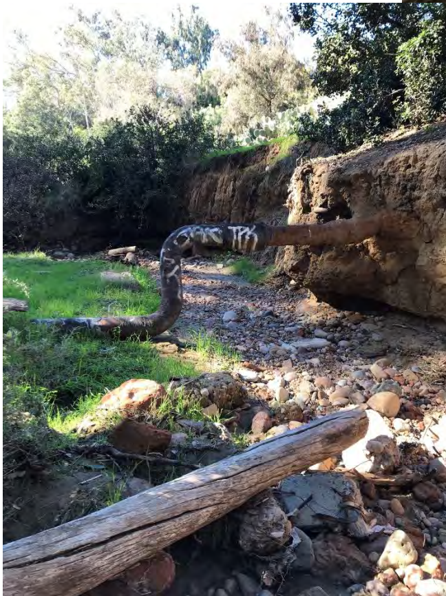
Photo 1.14: Looking south from 1.13 at location where creek has eroded soil that supported this sewer line.
