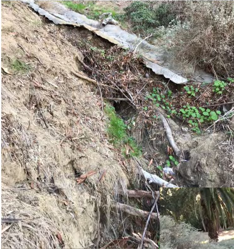
Photo 3.3: The end of the concrete which obviously does not carry the majority of the water from above. Water descends down in a chaotic manner beside it.
