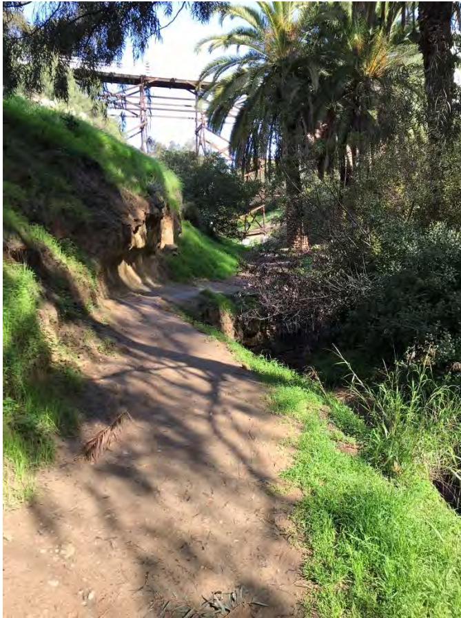
Photo 1.9: Looking north up canyon past the Canary Island palms in Photo 1.8, with the Quince Street Pedestrian Bridge in the background. The drainage is undermining the soil beside the trail and will soon cause the collapse of the trail in this section.
