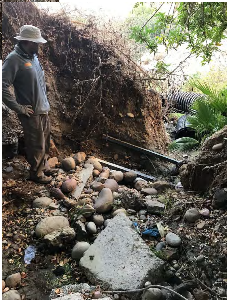
Photo 1.4: The erosional hole that has been carved by the broken pipe. Debris including pieces of broken pipe were visible.
