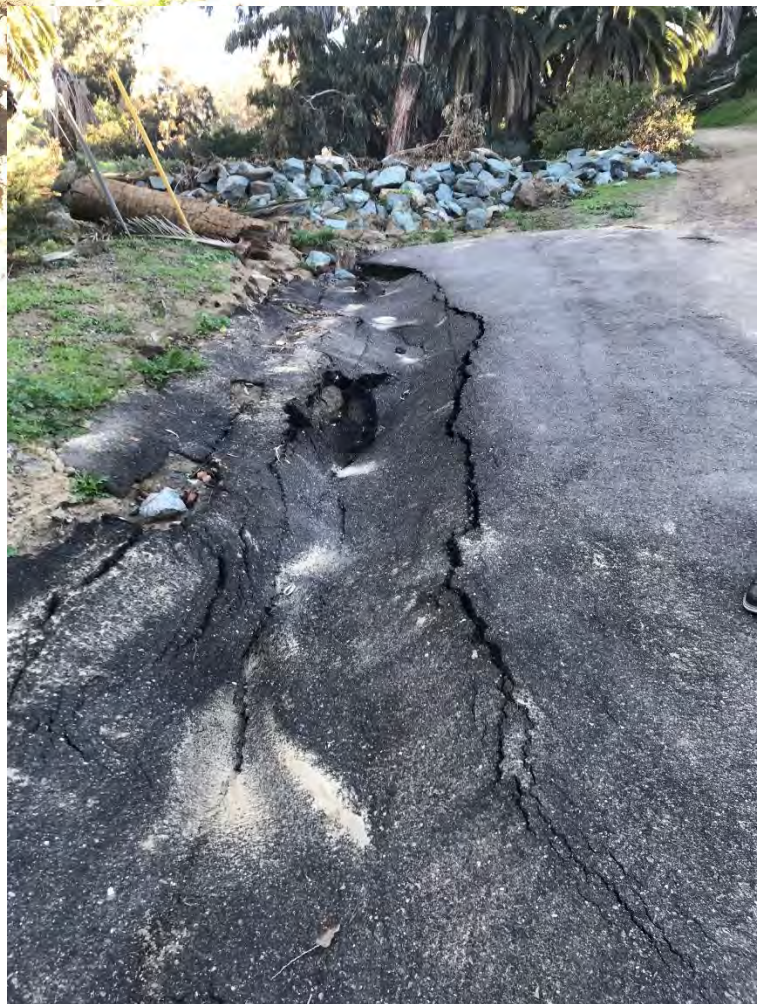
Photo 1.31: looking east towards the riprap holding back the sediment-filled detention basin. Water has undermined the asphalt of the controlled access at the western end of the canyon.
