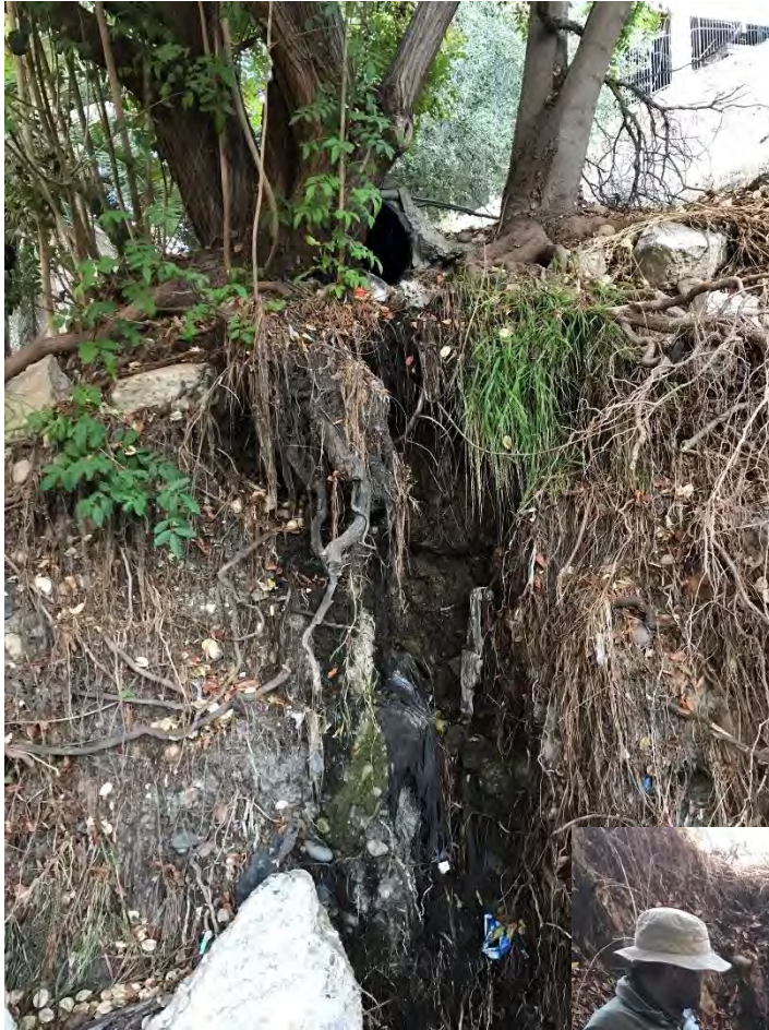
Photo 1.3: The broken corrugated plastic SD pipe opening is visible at the base of the tree trunks (upper middle of photo). Water has carved a large hole in the canyon floor.
