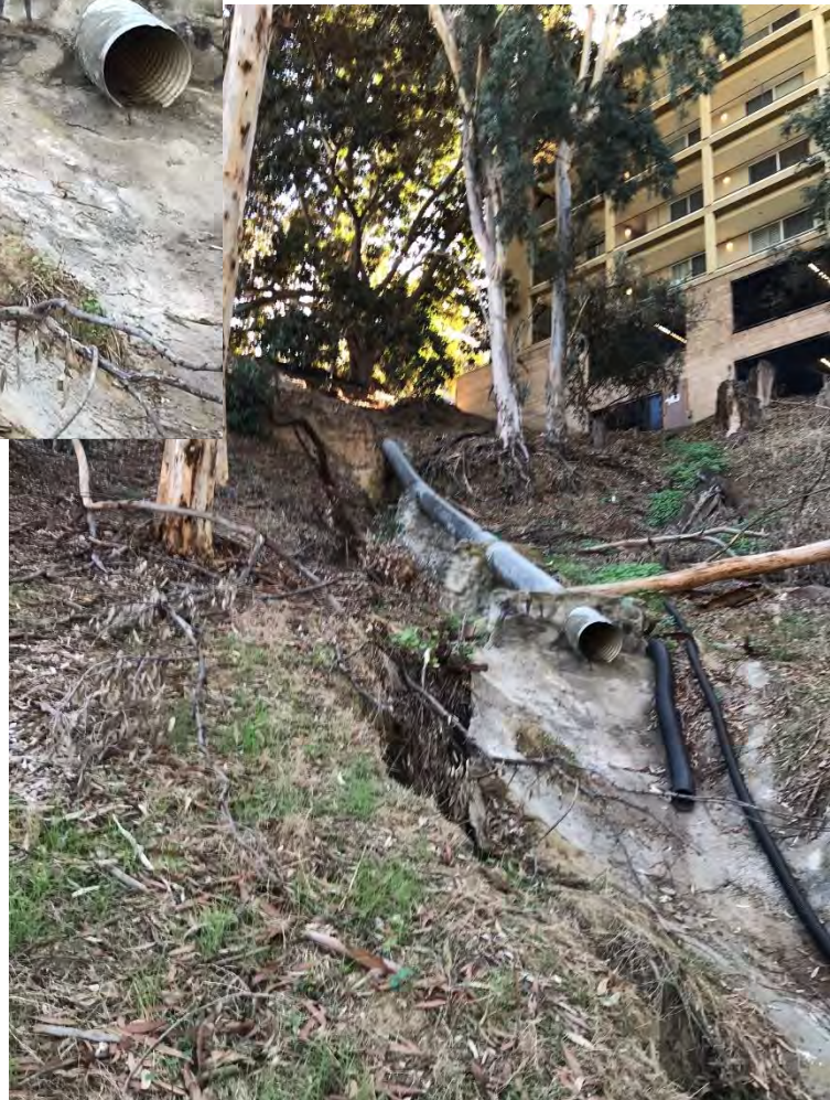
Photo 3.2: Black plastic pipes carry water from the building to the right down to the concrete.
