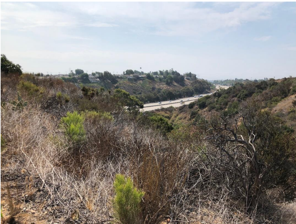
Photograph of the MHPA south of Birmingham Way with I-805 Photograph taken facing south from the generator facility on August 16, 2021
