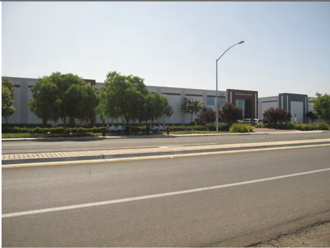
1. Concrete tilt-up industrial buildings
