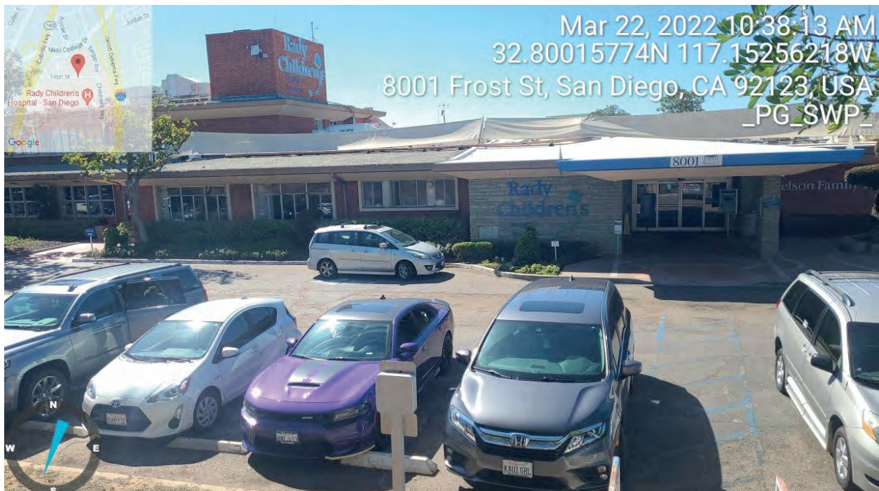
View southwest toward the access point of the Nelson Pavilion located on the northwest portion of the Project boundary.
