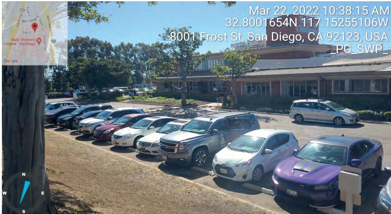
View southwest toward the Nelson Pavilion located on the north portion of the Project boundary.
