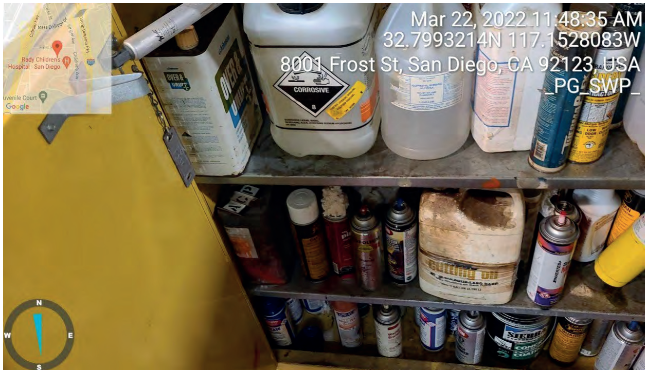
View south in a room located on the second floor of Building 12 on the west portion of the Project boundary. Chemicals and aerosols are stored in locked container.
