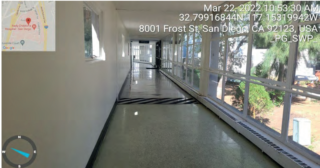
View northwest inside a hallway within Building 12 located on the west portion of the Project boundary.
