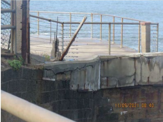
View looking South, upper area of wall failing. Northern view of the collapsed fence post with fence propped up.
