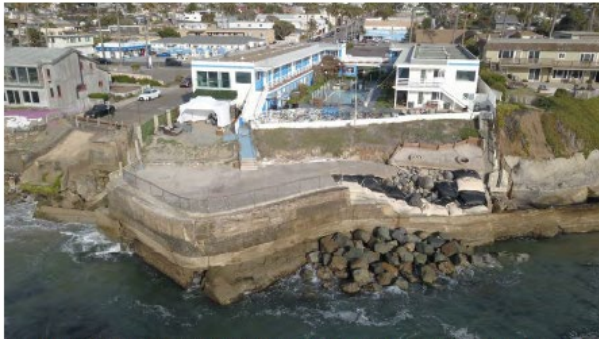
Crack and cave in sea wall is directly below cracking recently appeared in deck. This photo 4-2021.
