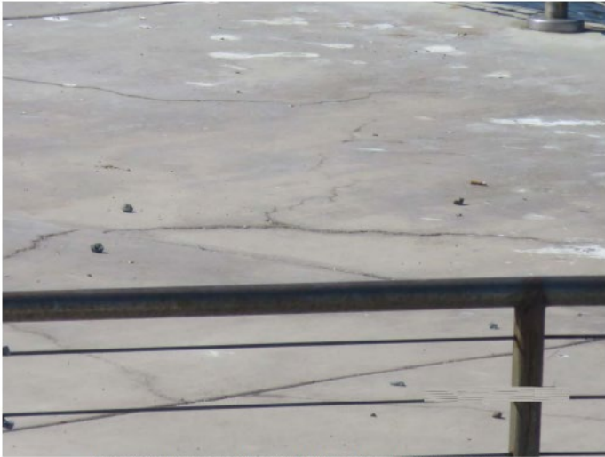
Photo showing larger area. May signify shifting of the underlying cement layers.
