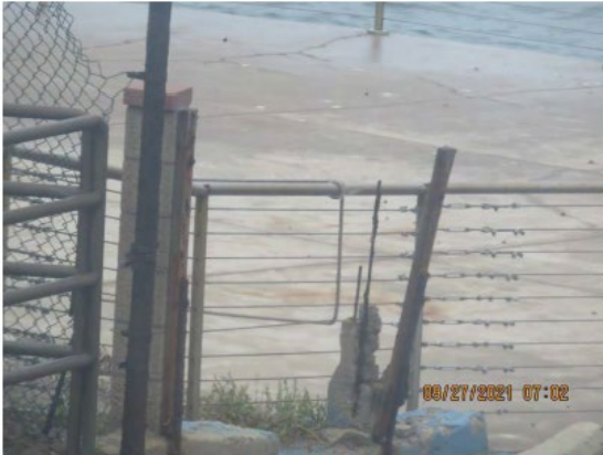
This fence post has broken directly over one of the voids, and the fence is propped up with a stake.
