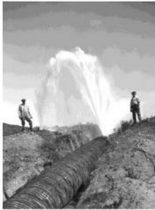
Wooden pipe often failed
