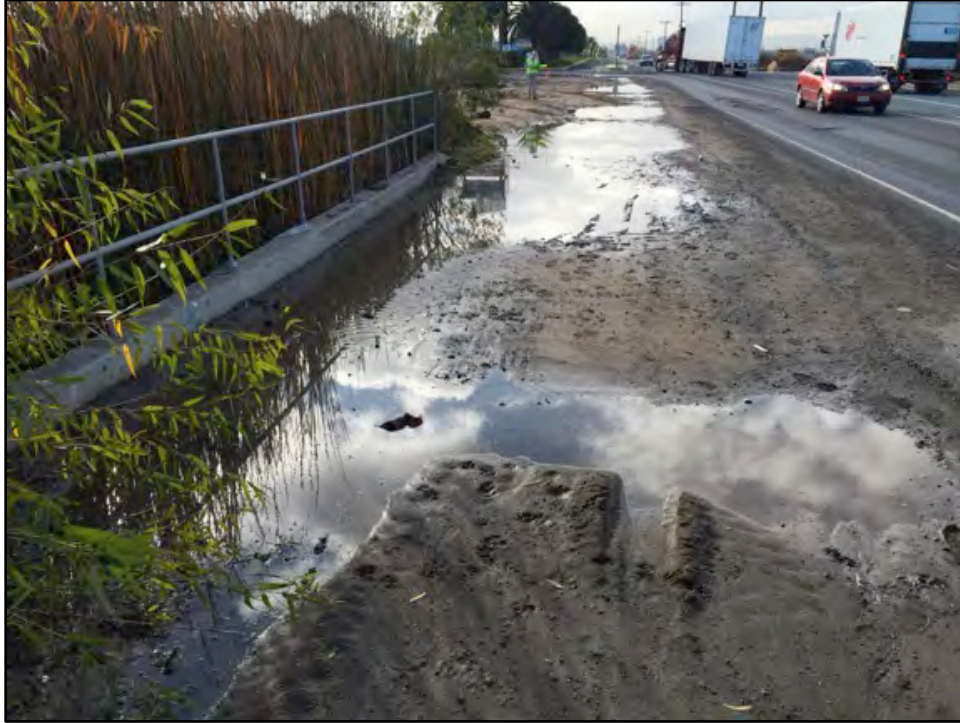
Photograph 1. View of road rut Basins 8a-c northeast of intersection of Airway Road and La Media Road (facing south; taken December 18, 2014). One unidentified, female Branchinecta fairy shrimp was detected within Basin 8a on January 3, 2015.
