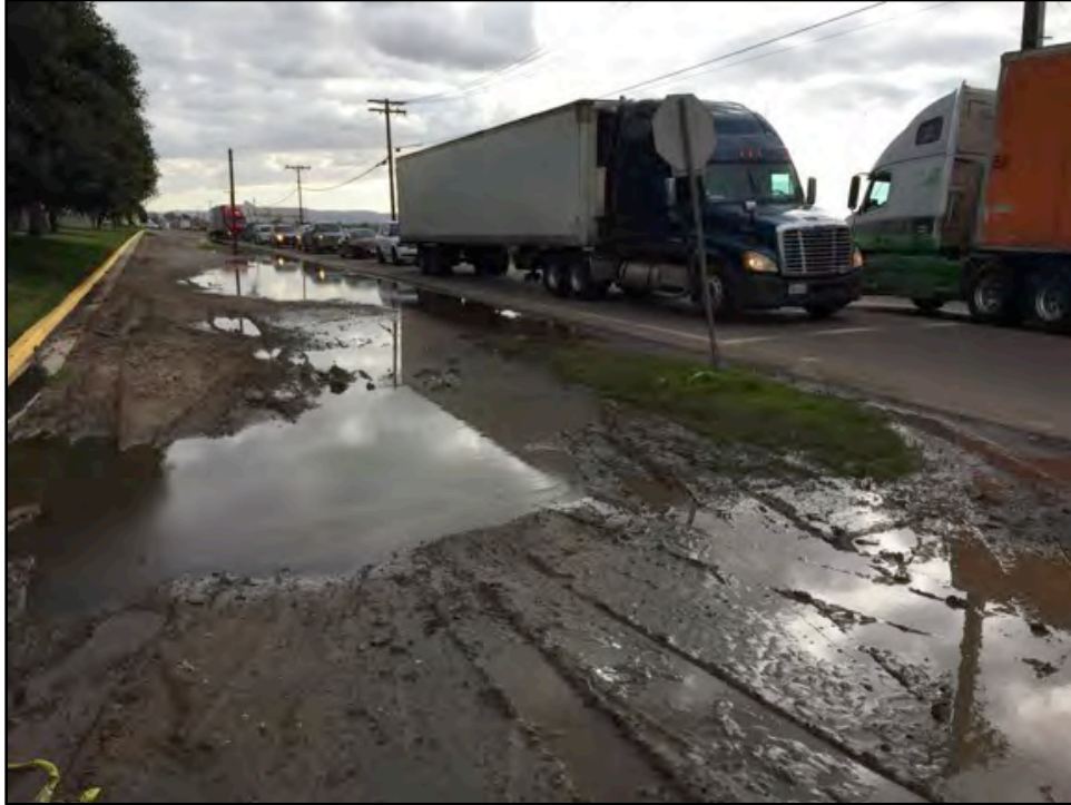
Photograph 3. View of road rut Basins 44a-e southeast of intersection of Airway Road and La Media Road (facing south; taken December 18, 2014). Basin 44a in foreground was partially filled by adjacent irrigation runoff throughout wet season survey.
